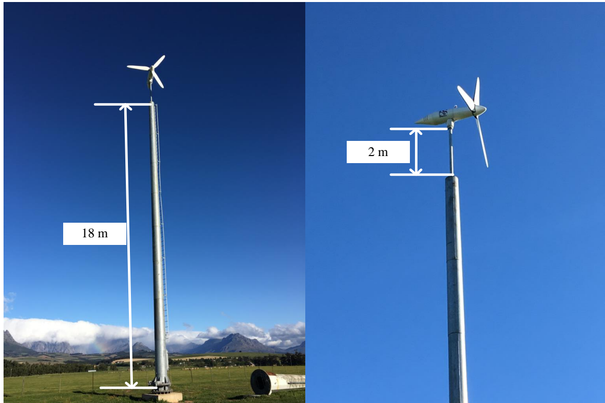
Figure 5.15: 2.2 kW downwind turbine at the Stellenbosch University Mariendahl small wind turbine testing facility.
