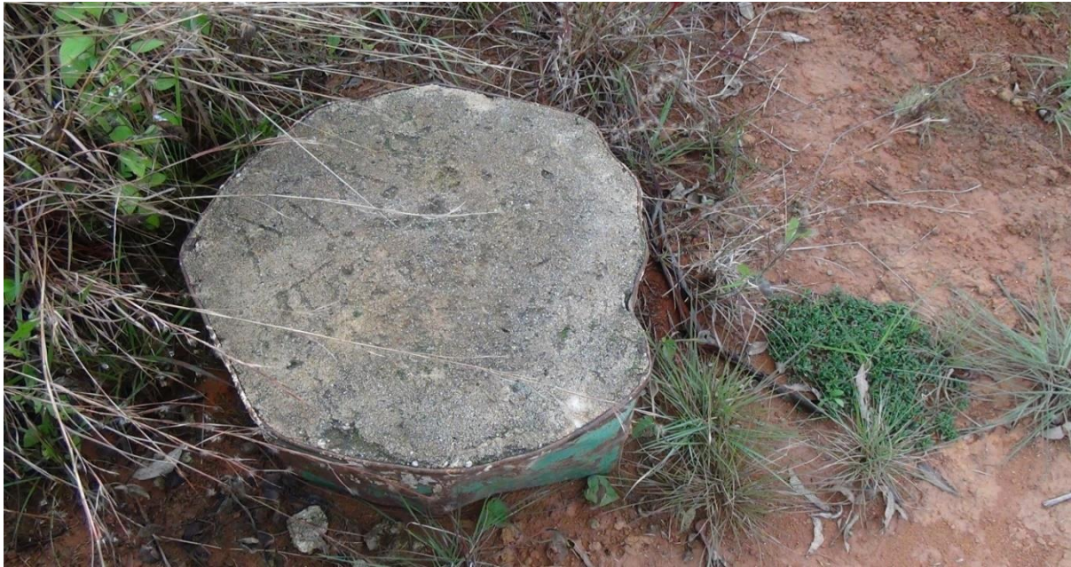
Figure 12: A barrel filled with cement as a sign of boundary. 123
