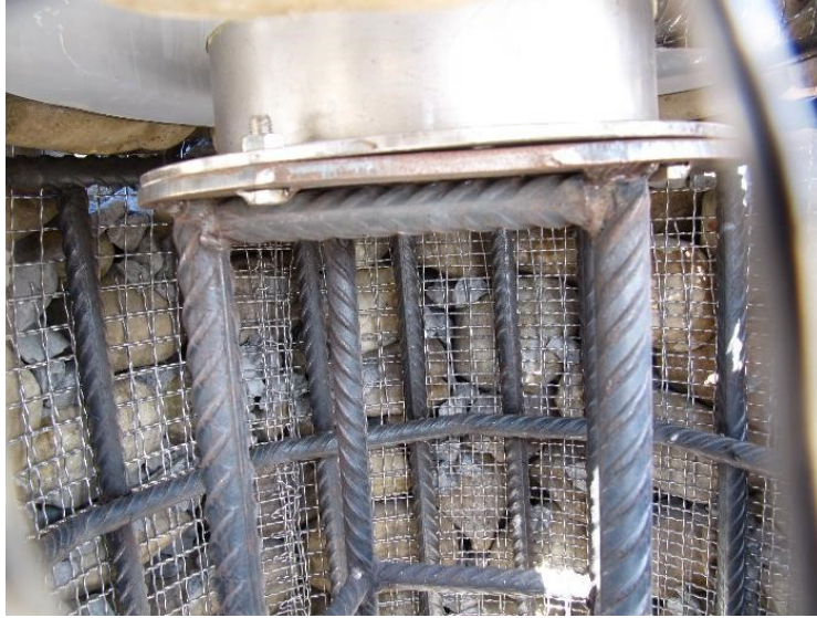
Figure 3.10: Inner view of the air outlet distribution structure
