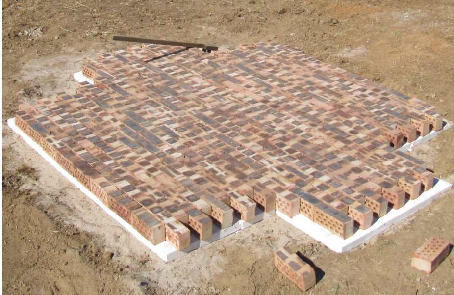
Figure 3.4: Base insulation beneath the thermal storage facility under construction
