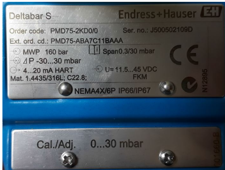
Figure E.1: Name plate of the Endress and Hauser pressure transducer
