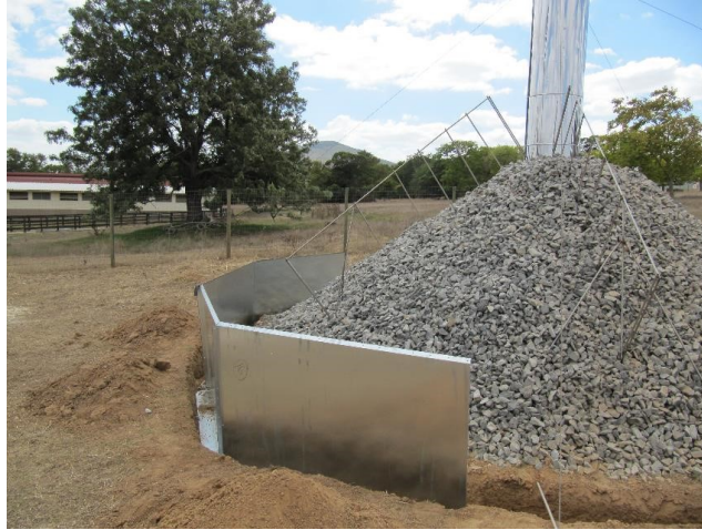
Figure 4.5: Installation of the walls in trenches
