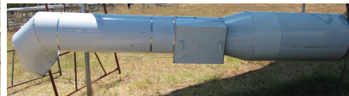
(b) Hot air ducting
