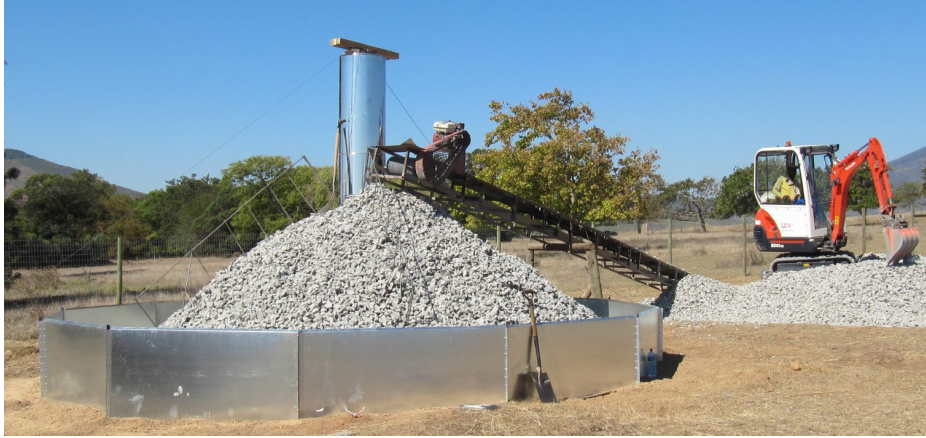
Figure 4.6: Stacking of the rocks by using a conveyor belt and a small excavator
