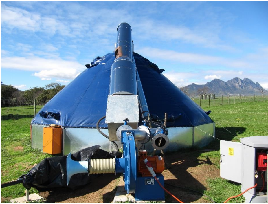
Figure 4.3: Operating TES in a charging state
