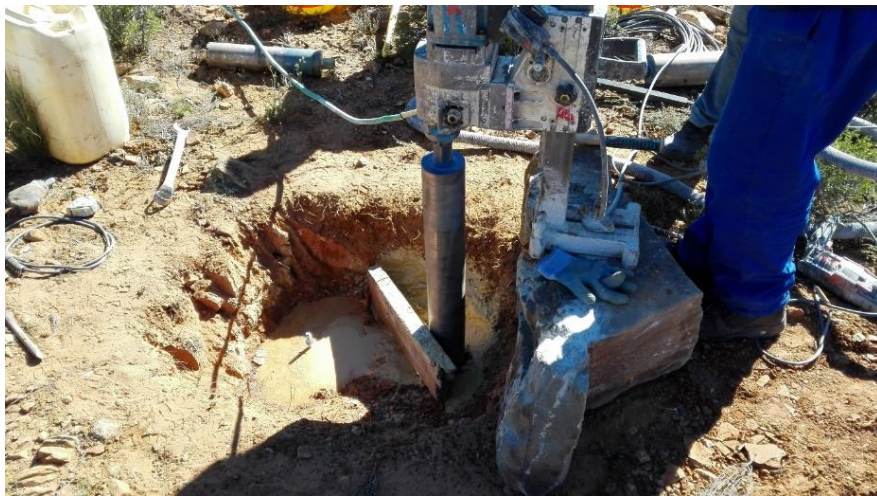
Beginning of drill run
