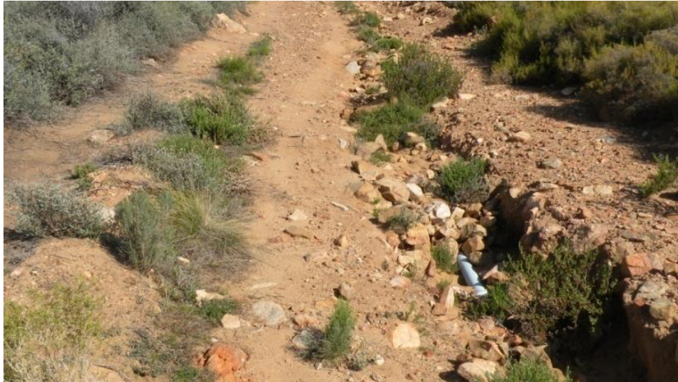
Figure 6-1: Access road showing erosion
