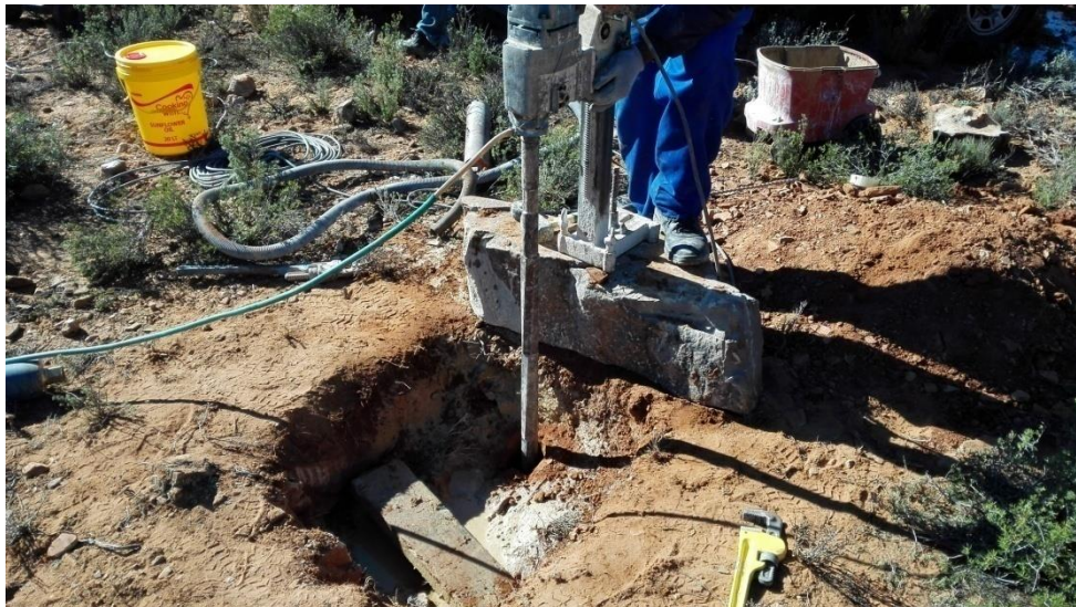
Figure 3-3: Drilling in progress
