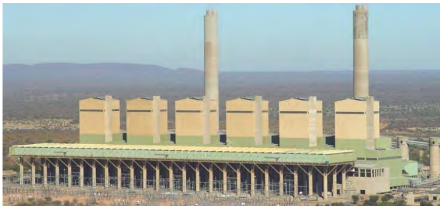
Figure 2.1: Matimba coal-fired power station (Pretorius, 2012).
