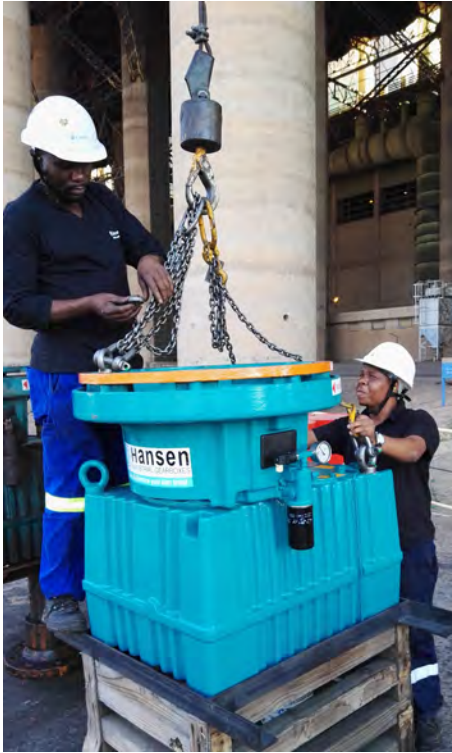
Figure G.16: Connecting the lift to the gearbox on the ground.
