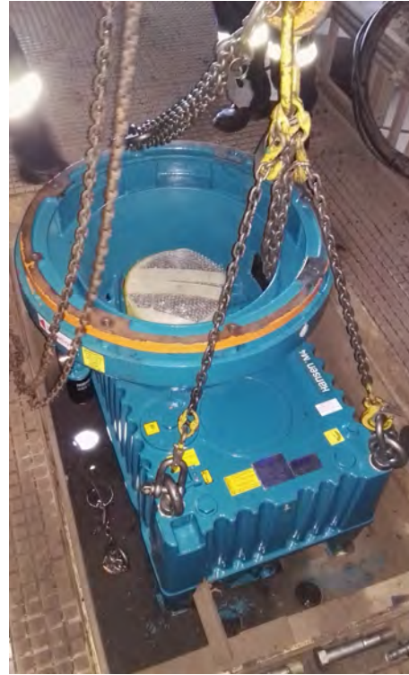
Figure G.17: Gearbox being lowered into position in the ACC.
