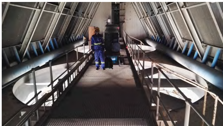
Figure G.19: Installation complete.
