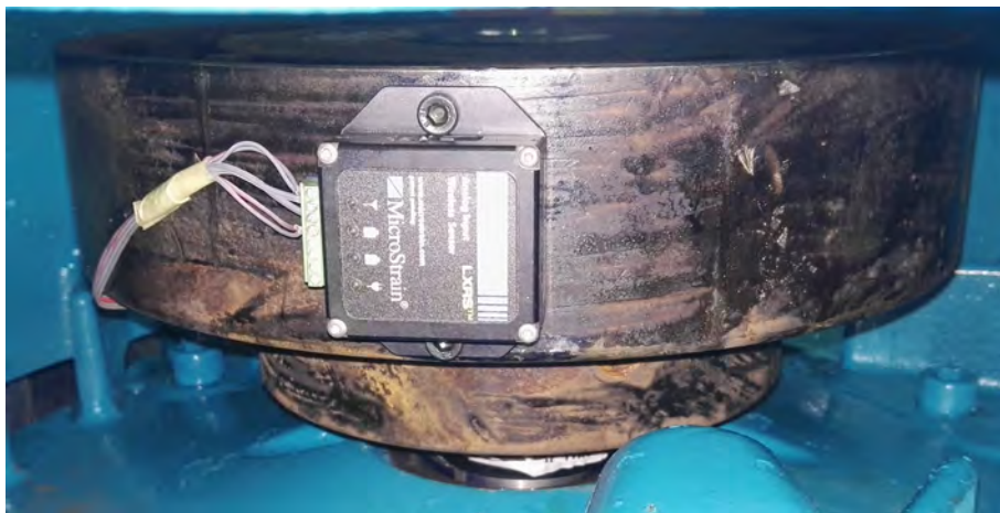
Figure G.12: SG-Link-LXRS installed onto high speed coupling with free hanging connecting wires.
