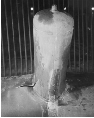
Figure 5.3: Typical failure of 90 degree special (Sang et al. (2002)).
