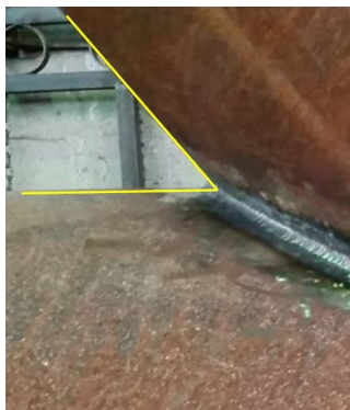
(a) Prior to pressure test.
