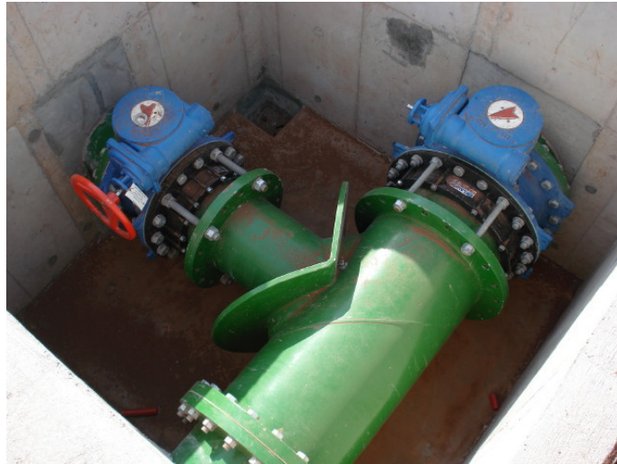
Figure 2.13: Two plate crotch plate installed at Sishen Mine (Aurecon).
