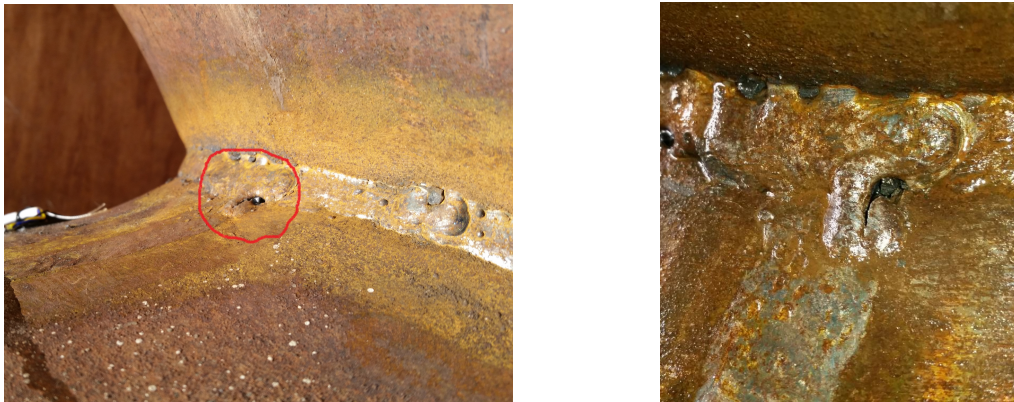
Figure 5.2: Small crack in acute corner.
