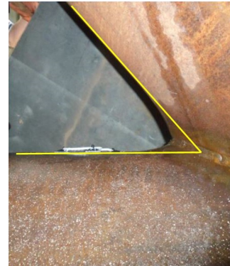
(c) Permanent deformation after pressure test.
