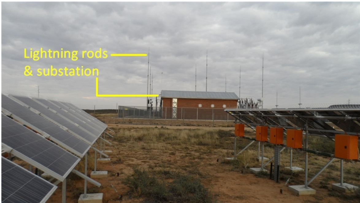
Figure D.2: Substation and lightning rods which cast a shadow.
