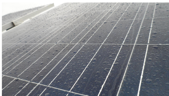
(a) Coated module surface after rainfall.
