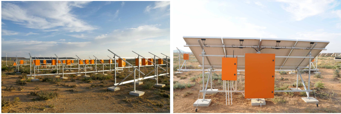
(a) Stationary PV module structures. (b) Battery bank after phase 1 installation.
