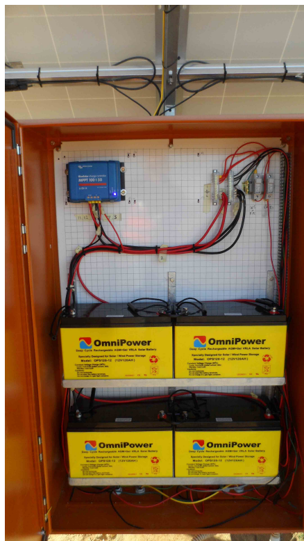
(a) Batteries and MPPT charge controller.
