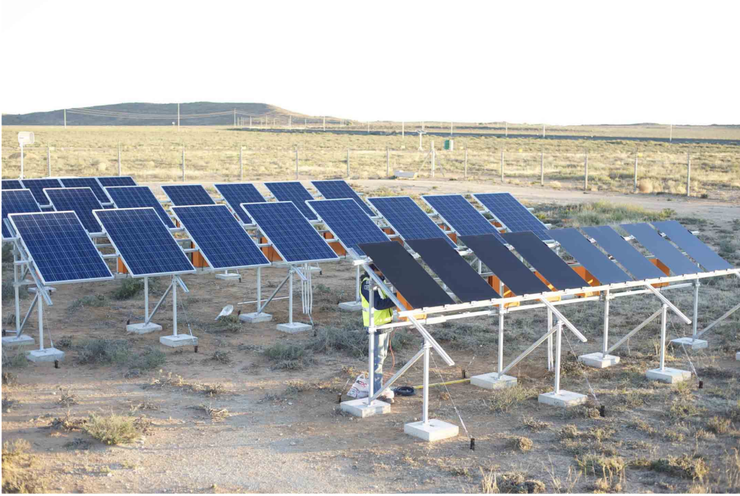
Figure 3.5: Image of PVRF and the three stationary north facing PV module rows, with thin-film modules in front and the polycrystalline modules behind.
