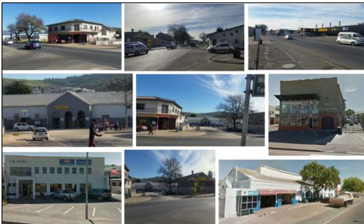
Photo 4: The structural condition of Du Toit station precinct
