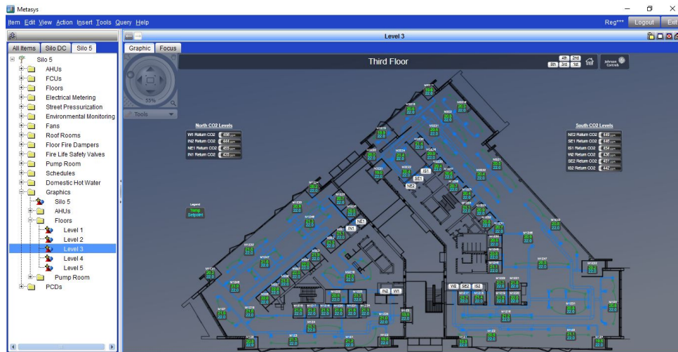
Figure 3.13: BMS user interface: Level 3 floor layout graphics view showing temperature, pressure and CO_2 readings and set points
