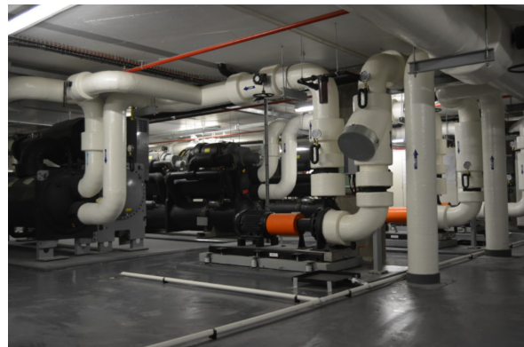
Figure 3.2: District cooling plant chillers and pumps
