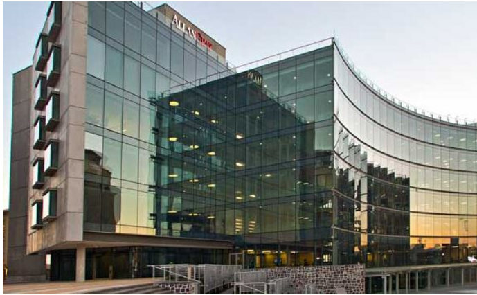
Figure 2.3: No. 1 Silo building [9]
