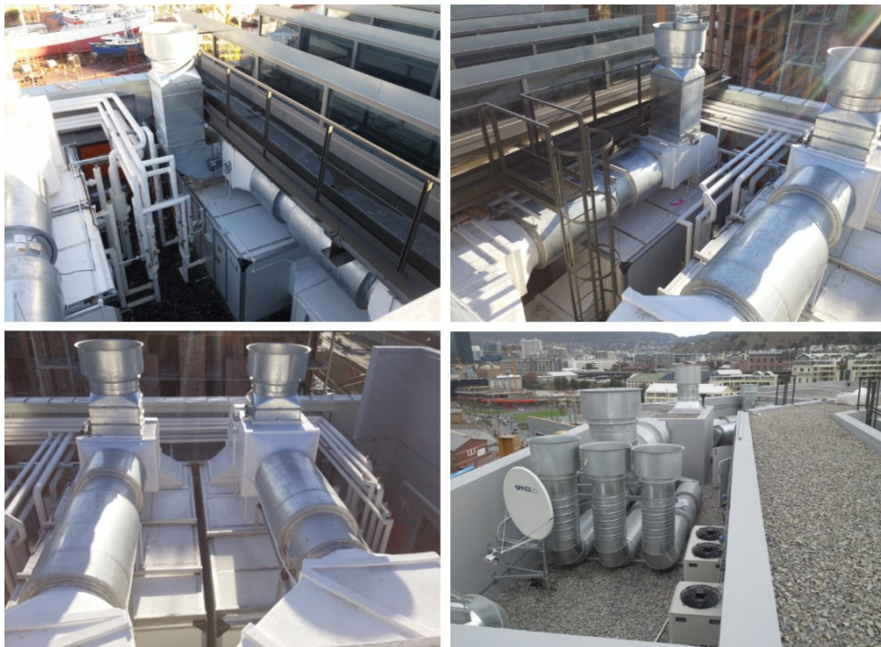
Figure 3.5: Silo 5 rooftop plantrooms
