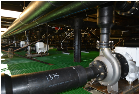
Figure 3.1: District cooling seawater pumps at the jetty
