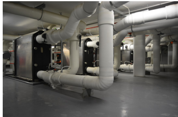
Figure 3.4: District cooling plant heat exchangers
