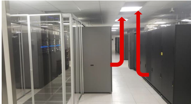
Figure 2.14: Data centre hot aisle [37]
