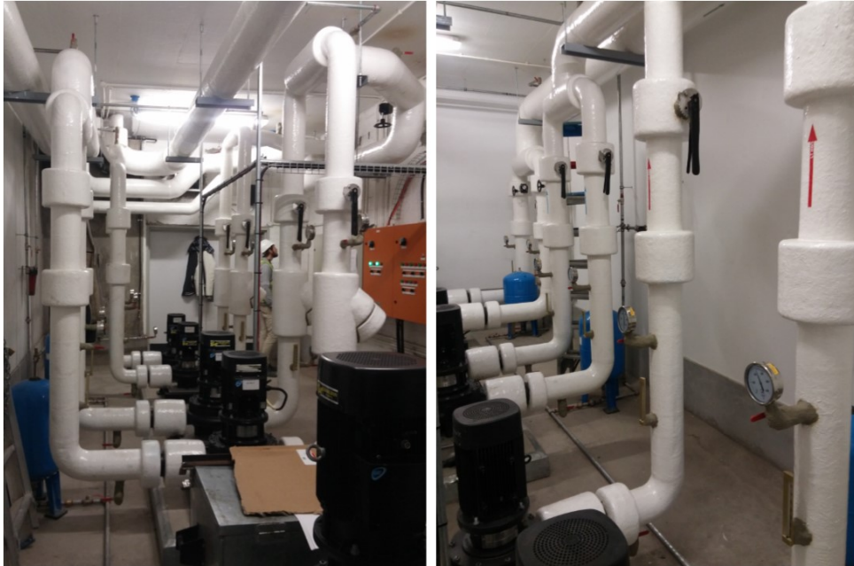
Figure 3.11: Silo 5 basement plantroom with secondary pumps and piping systems
