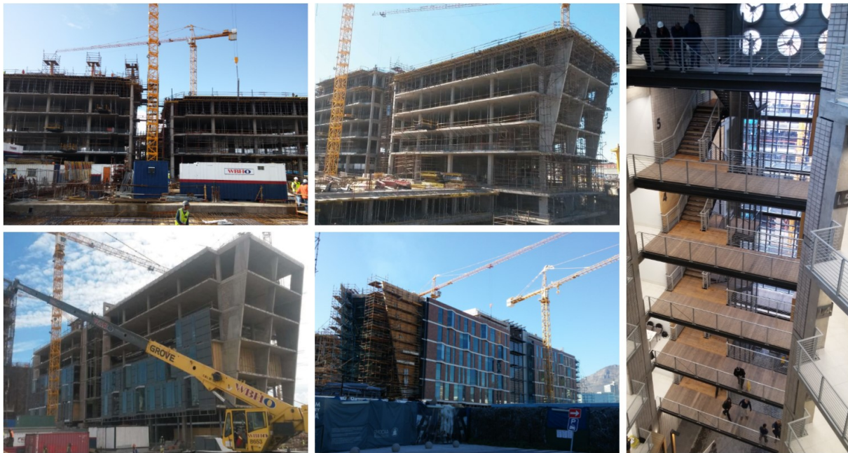
Figure 1.5: No. 5 Silo construction
