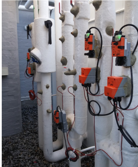
Figure 3.8: Belimo Energy Valves installed on the return side of PCW, CHW and HHW pipes at one of the Silo 5 rooftop AHUs
