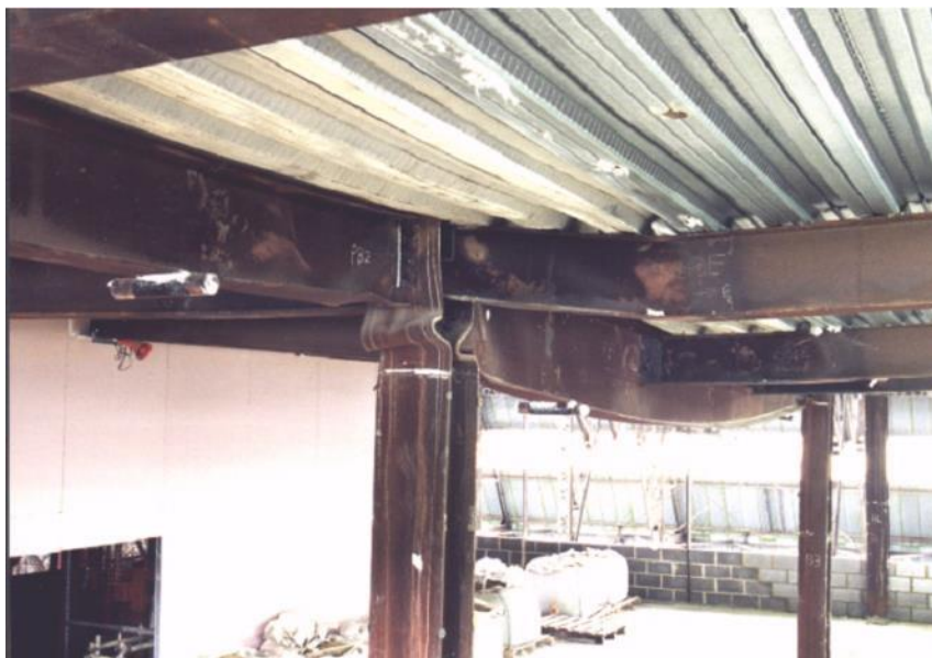
Figure 2.5: Failed column and beams at the Cardington fire tests (Lamont 2001)
