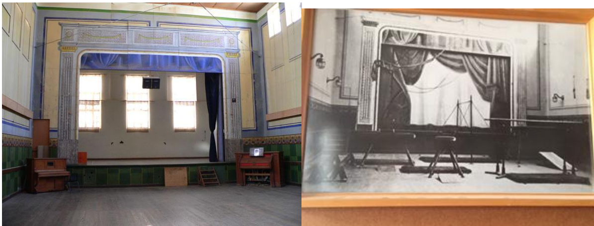
Figure 4.15: The restored and the original Turnhalle (Gym Hall) or Konzertsaal (Concert Hall). Notice the installed with gymnastics equipment, a balcony at the back, a stage in front, and a harmonium and piano on display. The kitchen at the back of the hall was able to cater for 300 people at a time in the adjoining dining room. Source: D.L. van Zyl (April 2015).
