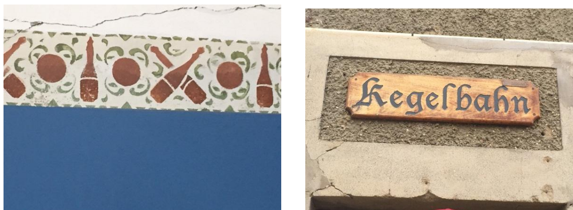
Figure 4.16: The original frieze on the wall of the skittle ally as well as the signboard above the entrance. Source: D.L. van Zyl (April 2015).
