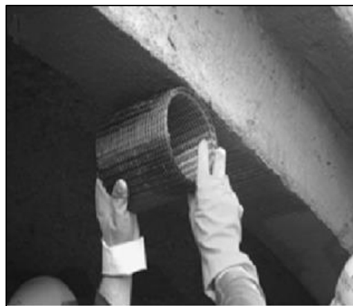
Figure A-12 Placing of the textile reinforcement (Schladitz et al., 2009)
