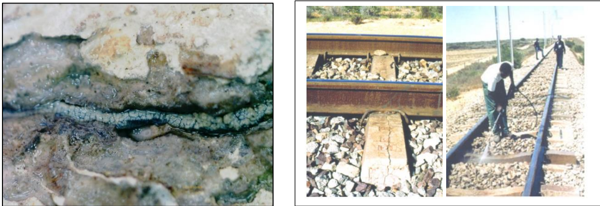
Figure A-10 Crack treatment, left: the crack width increased while a rigid epoxy has not changed in Good Hope Centre, Cape Town, and right: a part of treating the concrete sleepers with silane in the Sishen-Saldanha railway line, South Africa (Grabe and Oberholster, 2000).
