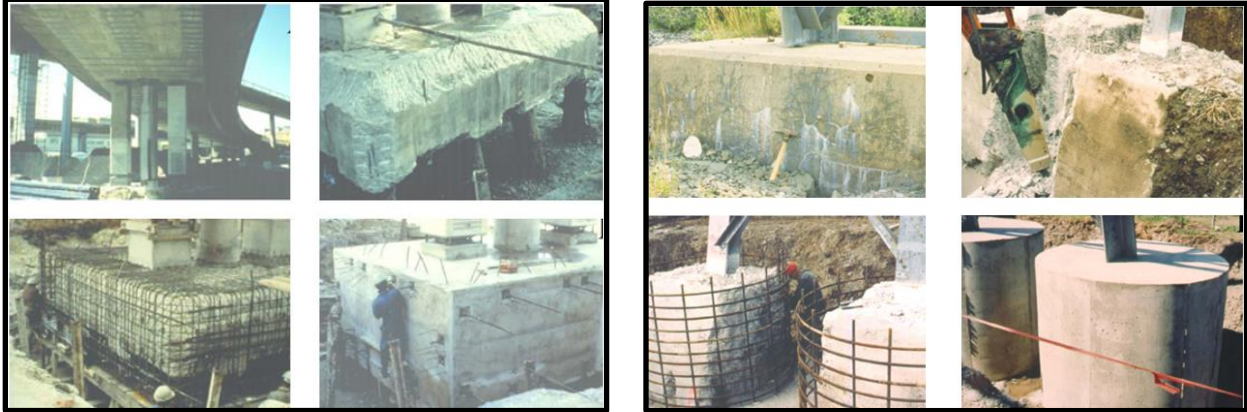
Figure A-13 Strengthening damaged by steel reinforced concrete, left: a highway structure affected by ASR in South Africa, and right: electricity tower concrete foundation affected by ASR in Quebec City, Canada (Fournier et al., 1991).
