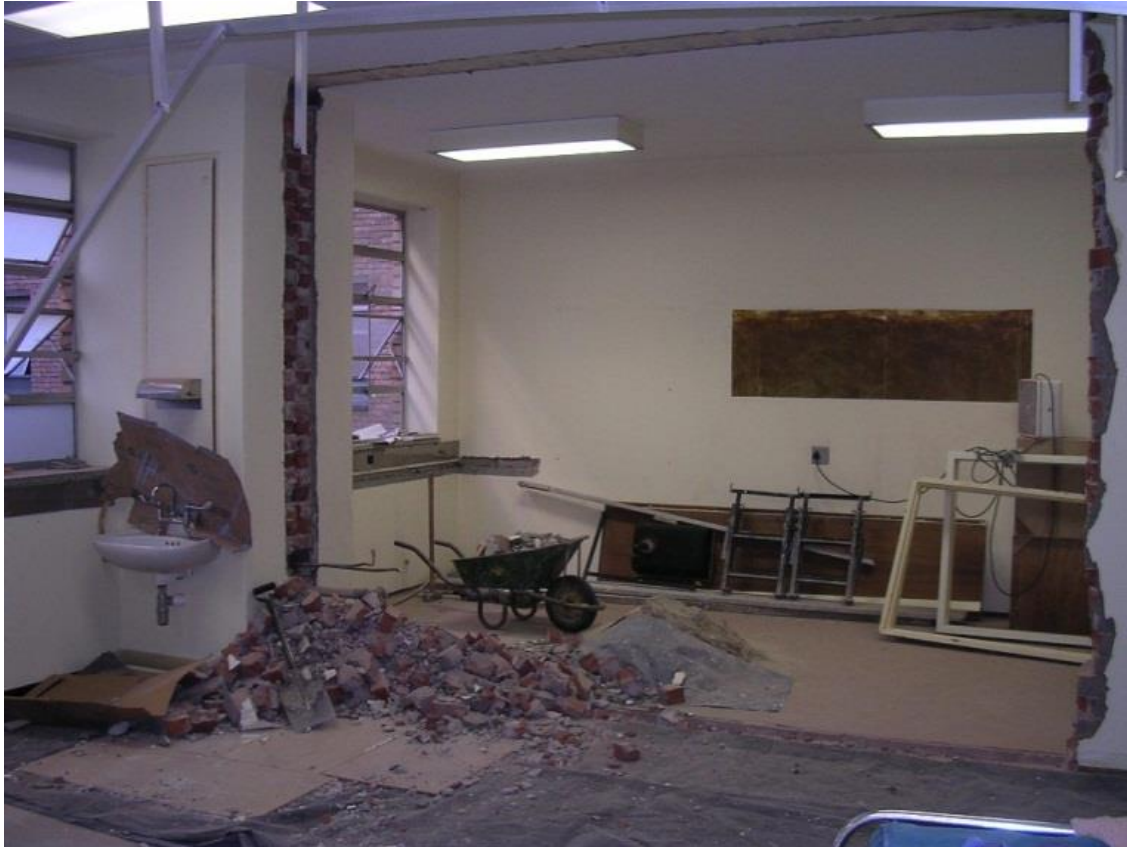
Photo 1: Construction of the Obstetric Critical Care Unit
