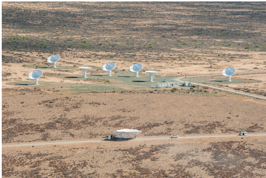
Figure 1.1: KAT-7, the precursor for MeerKAT shown in the background. The MeerKAT main reflector dish (centre front) is shown in transit during the setup stage [1].
