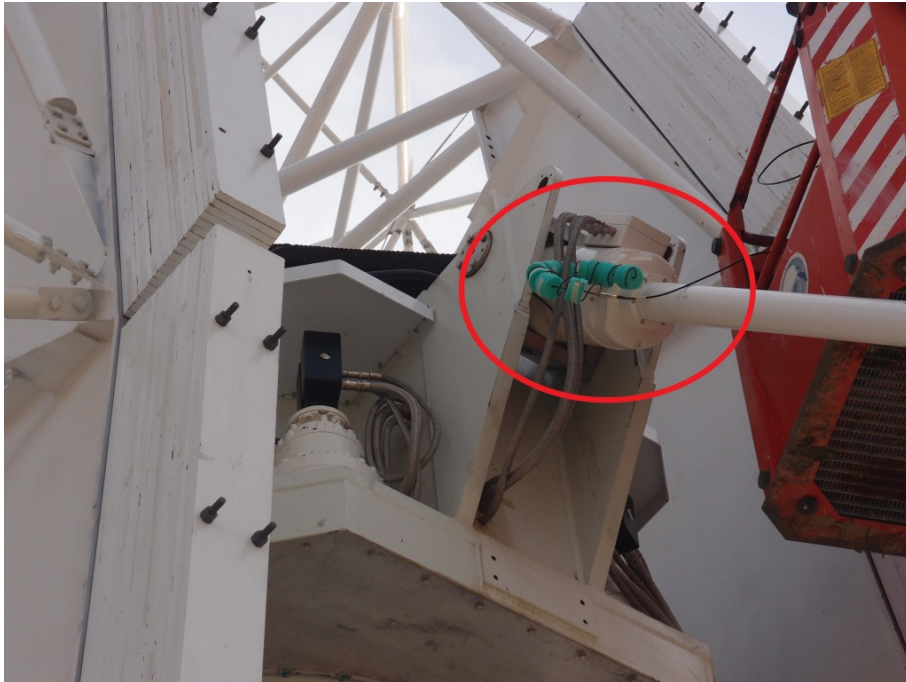
Figure 1.3: Implementation of an RC used on-site at M63
