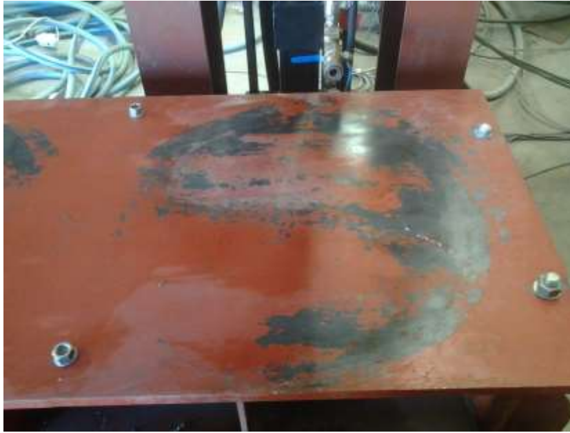
Figure 3- 39: Fixing of Platform to Support Beams to Increase Rigidity
