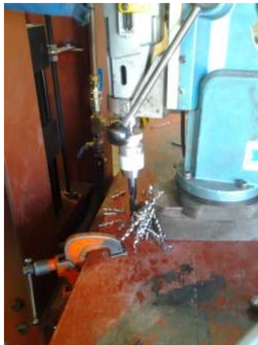
Figure 3- 38: Drilling of Holes through Platform and Support Beams
