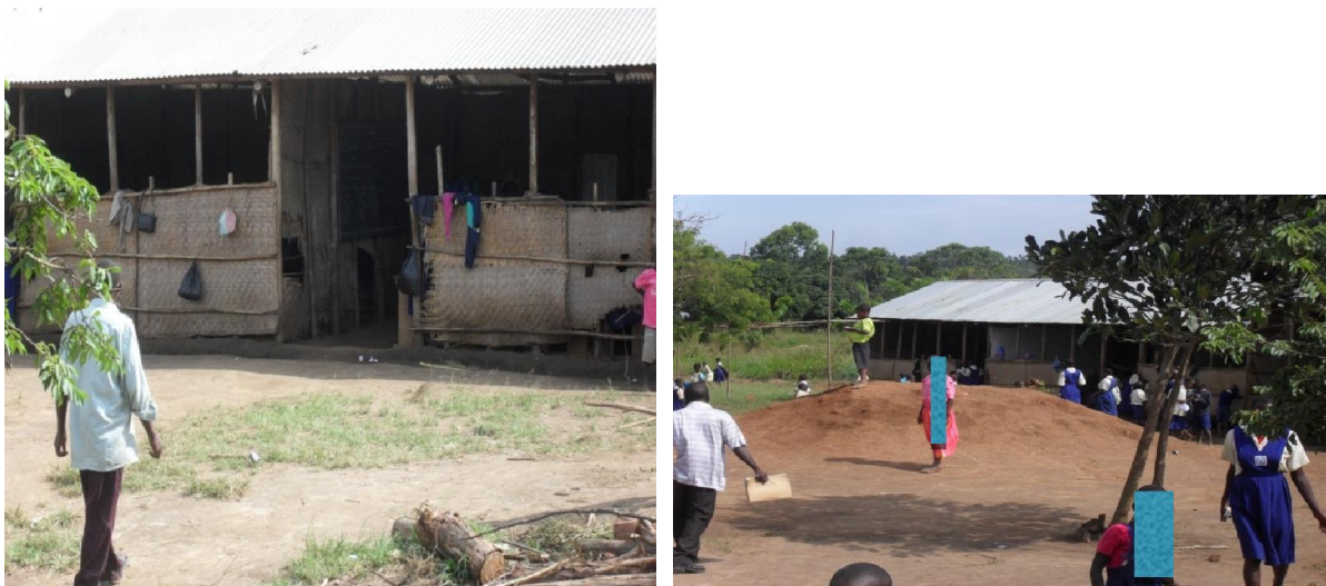
Figure 5A (1 and 2): Non-permanent school building (RakaiRP-C)
