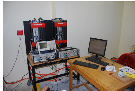
(d) Laboratory testing space with drives and RPSs.
