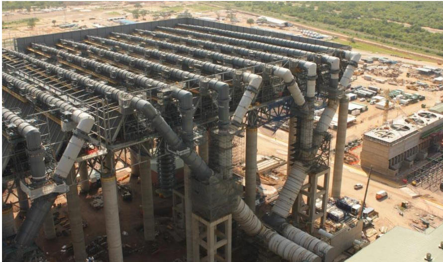
Figure 1.1 - Dry-cooled system of Medupi power station currently under construction.
