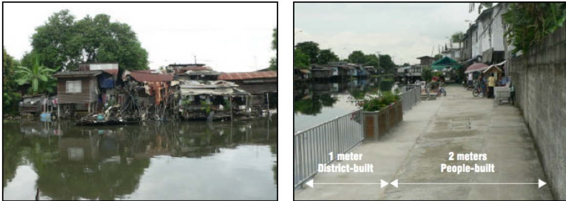
Figure 6.4: The Bang Bua Canal before (left) and after (right) upgrading
