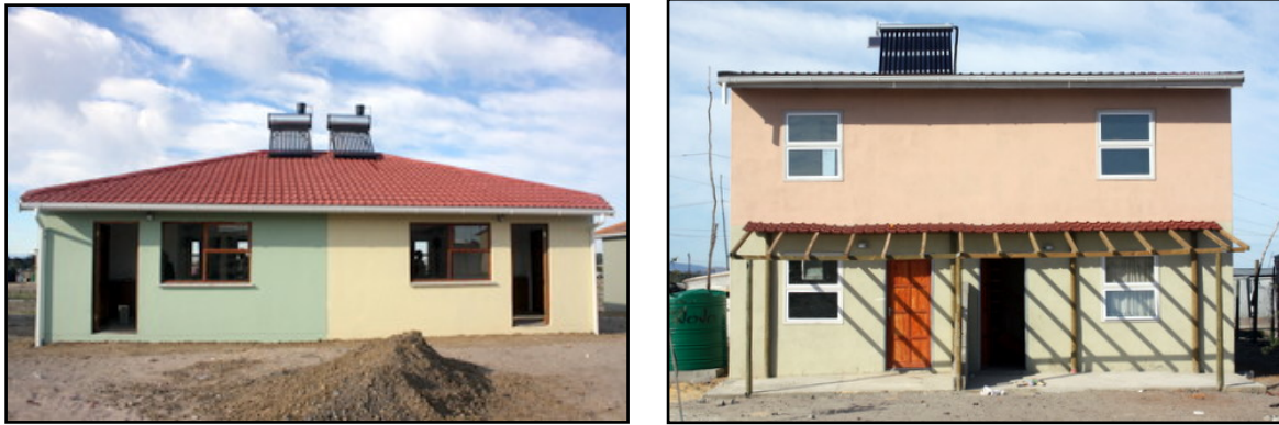
Figure 3.3: Witsand IEEECO™ semi-detached (left) and double story low cost housing units (right) Source: Photographs by Author (2012)
