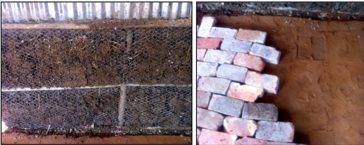
Figure 4.7: Installing Thermal Mass – Cob Wall under construction (left) and Recycled Brick Floor on moist clay (right)
