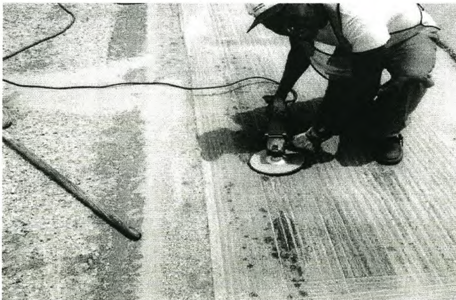
Figure 3.6: Grinding to smoothen Pad s3 (southbound lane)
