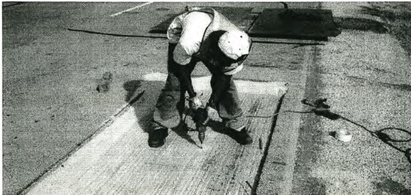
Figure 3.3: Drilling to install LPDs on Test Pad S3.
