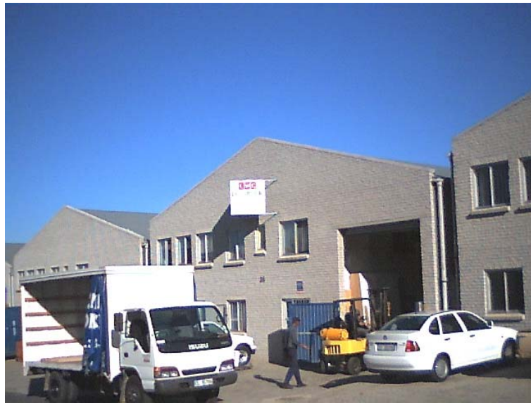
Figure 4.6: The roller door on the upper LWC factory floor, where raw materials are delivered.
