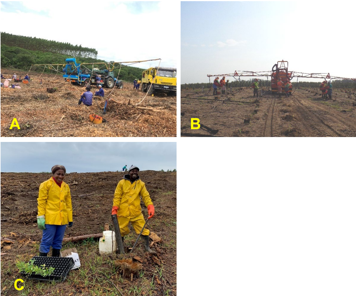
Figure 3.17 Planting operations. A- semi-mechanised 7-planter tractor drawn system. B- semi-mechanised 6-planter tractor drawn system. C- manual planting system.
