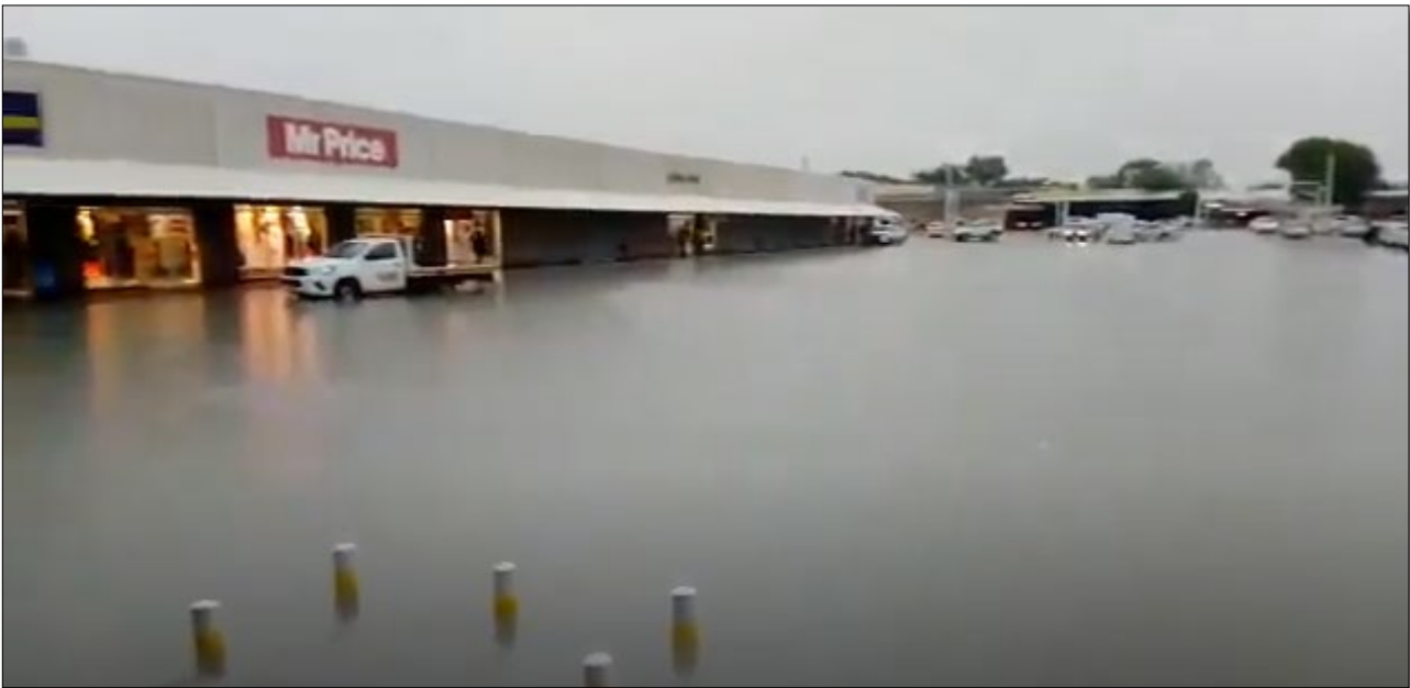
Figure 5.8: Business complexes heavily flooded during the rainy season in northern Namibia
