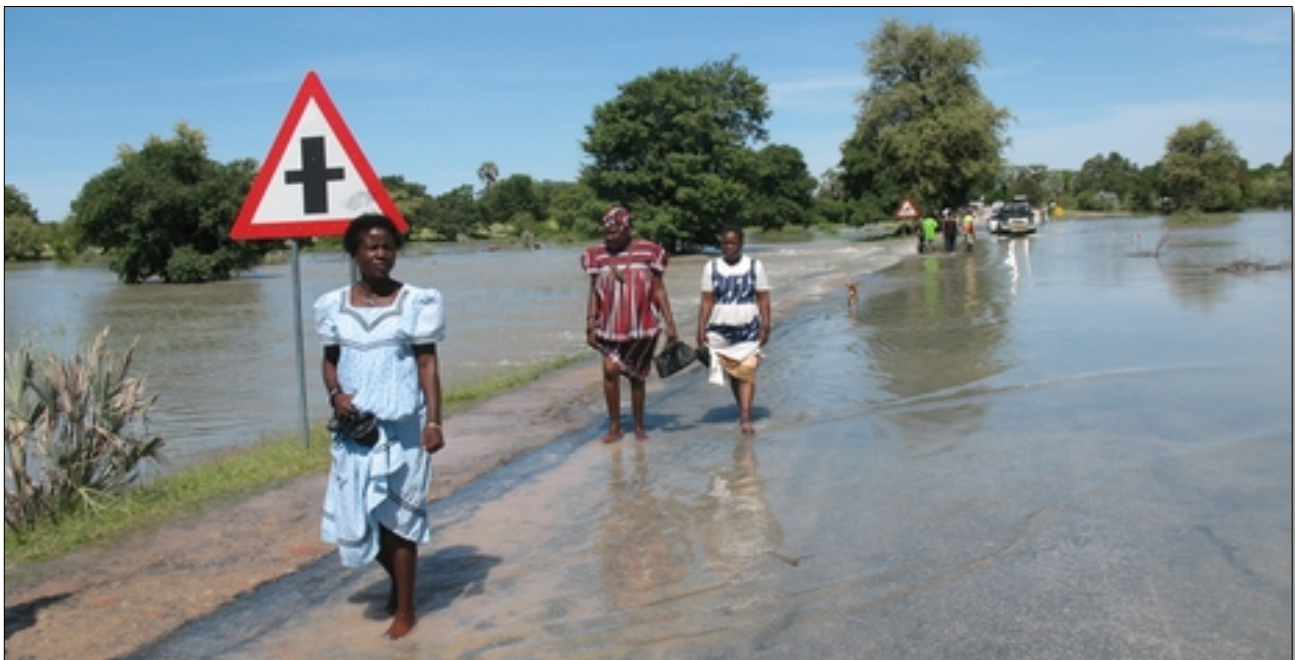
Figure 5.6: One of the local small bridges that has been submerged and passengers were forced to cross on foot
