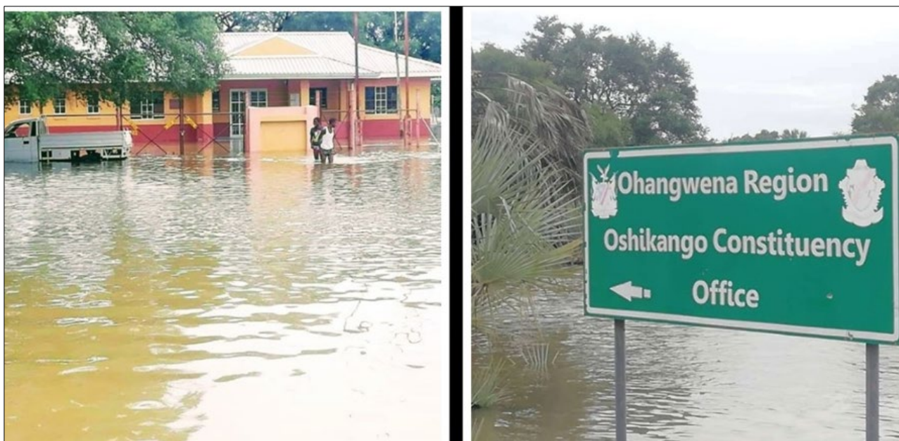
Figure 5.5: Impacts of Efundja on some of the government infrastructures of services – example of a constituency office flooded
