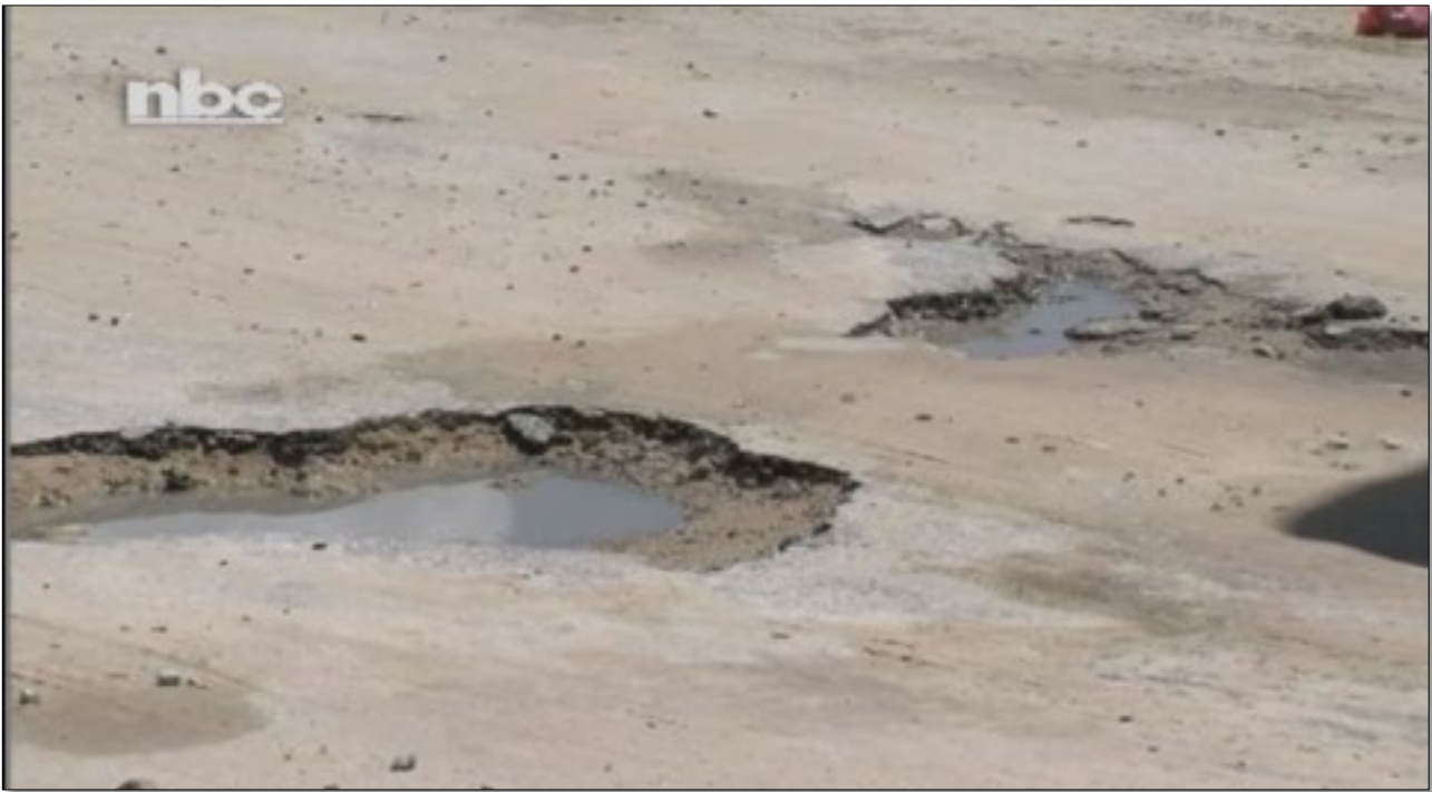
Figure 5.7: Road infrastructures damaged as a result of Efundja within the Cuvelai-Etosha basin
