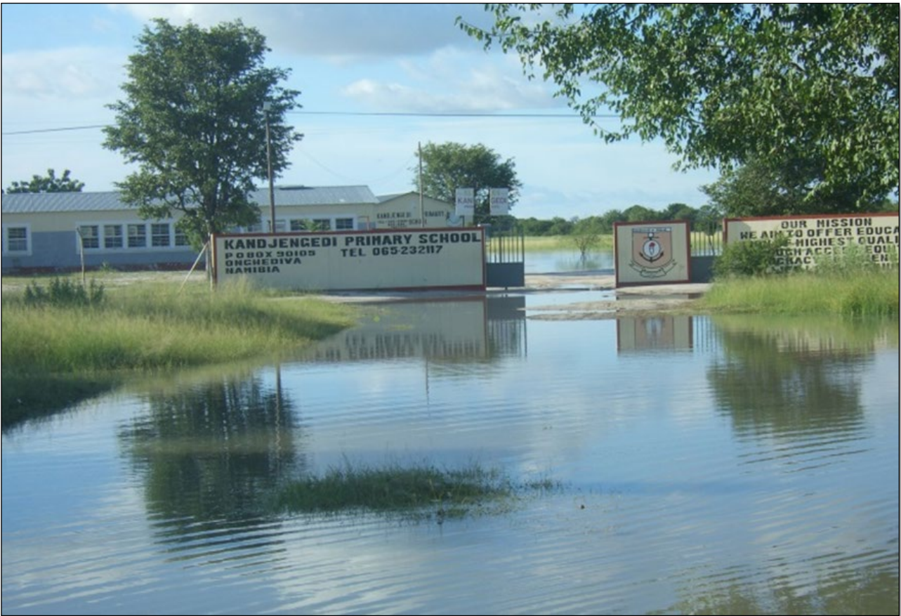
Figure 1.1: One of the schools routinely cut off by the Efundja
