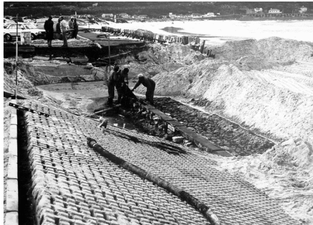
Figure 3.7 Sea walls in Fish Hoek A) Palisade sea wall constructed from wooden railway sleepers, 1980; B) Construction of a new (existing) seawall which was completed in 1982
