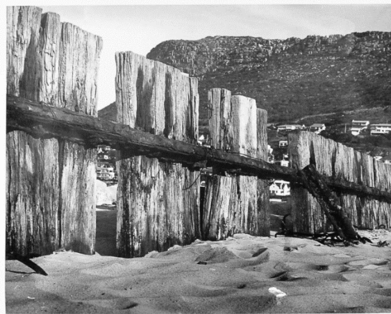
Figure 3.7 Sea walls in Fish Hoek A) Palisade sea wall constructed from wooden railway sleepers, 1980; B) Construction of a new (existing) seawall which was completed in 1982
