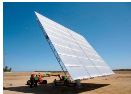
(b) 140 m 2 heliostat developed by Abengoa (Google Images)
