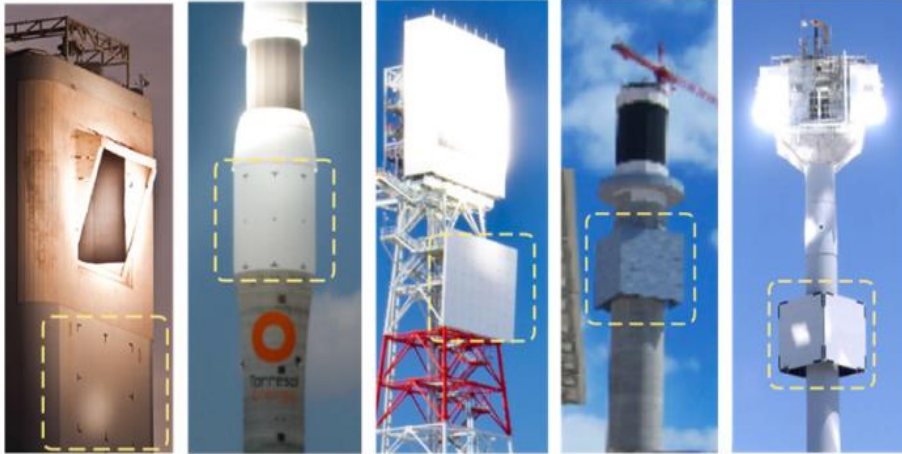
Figure 2.4: Different towers with their calibration target (Malan, 2014)
