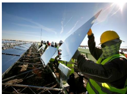
(a) 1.14 m 2 heliostat developed by eSolar (Google Images)
