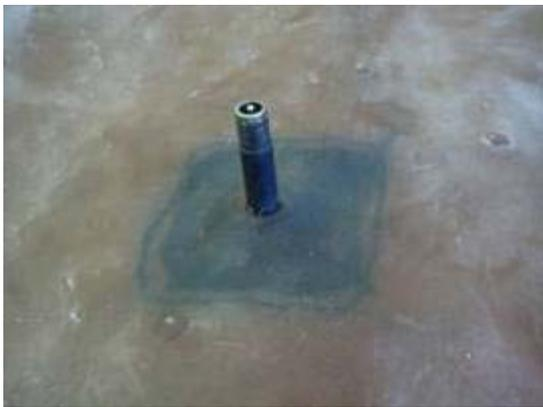
**Figure 36: Valve fitted on membrane**
