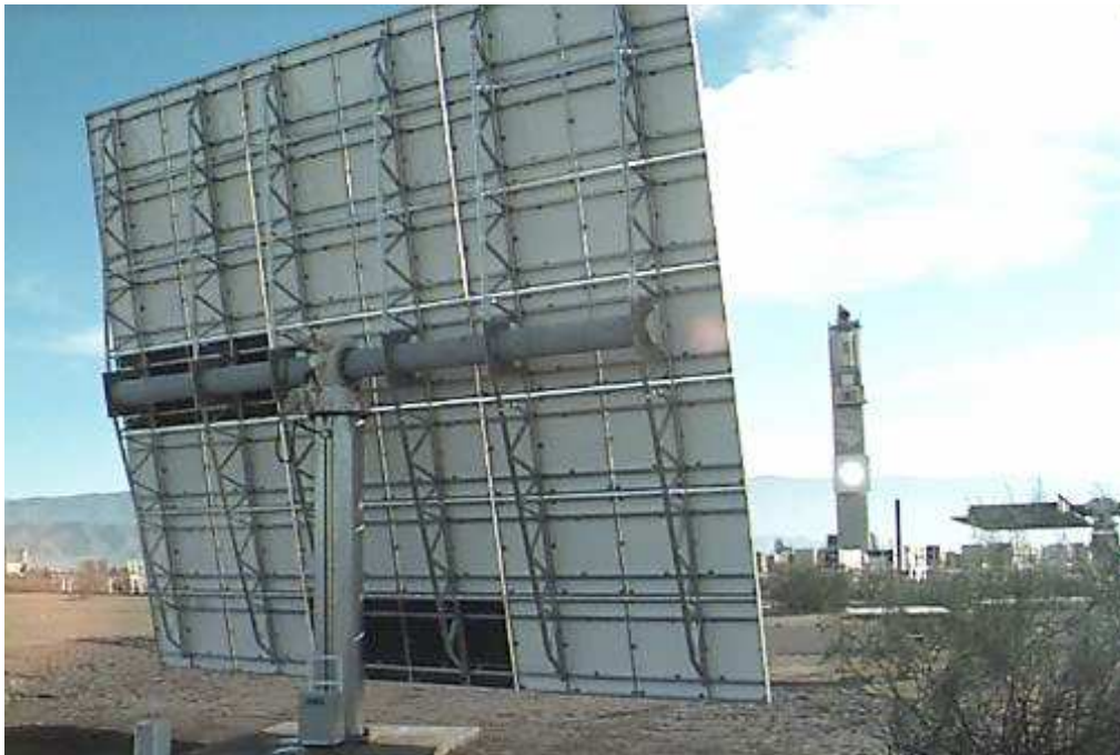
Figure 9: Support structure of a glass/metal heliostat (Colon 70).
