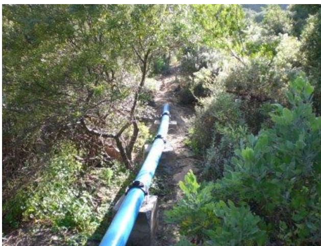
Figure G.8: Part of the above-ground pipeline and also showing the saddles holding the pipes to the concrete blocks.
