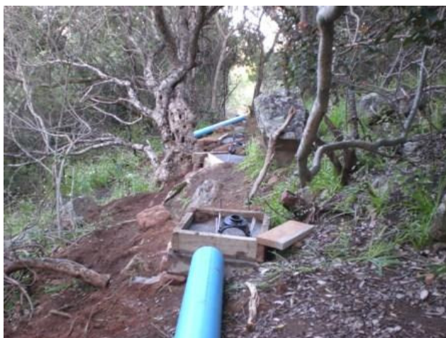
Figure G.7: Part of the above-ground pipeline during construction.
