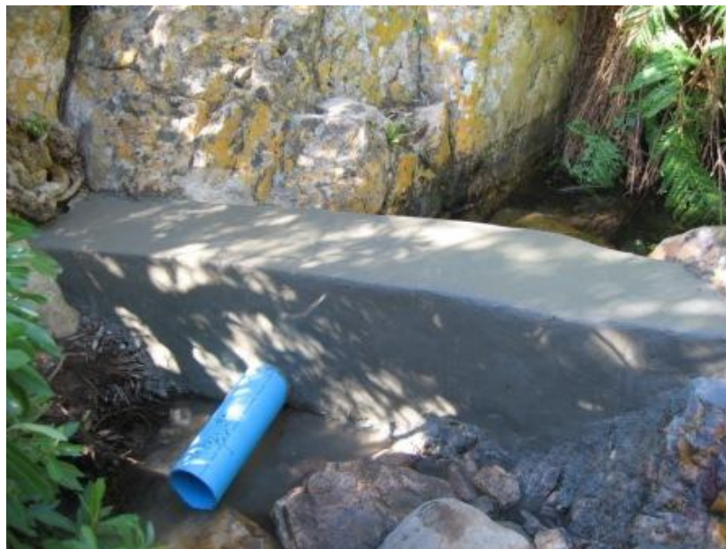
Figure G.3: The diversion weir just after construction.
