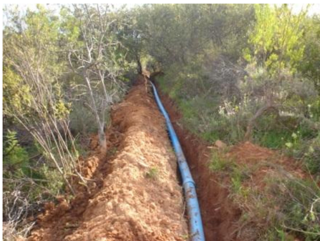
Figure G.6: The underground part of the main pipeline during construction.
