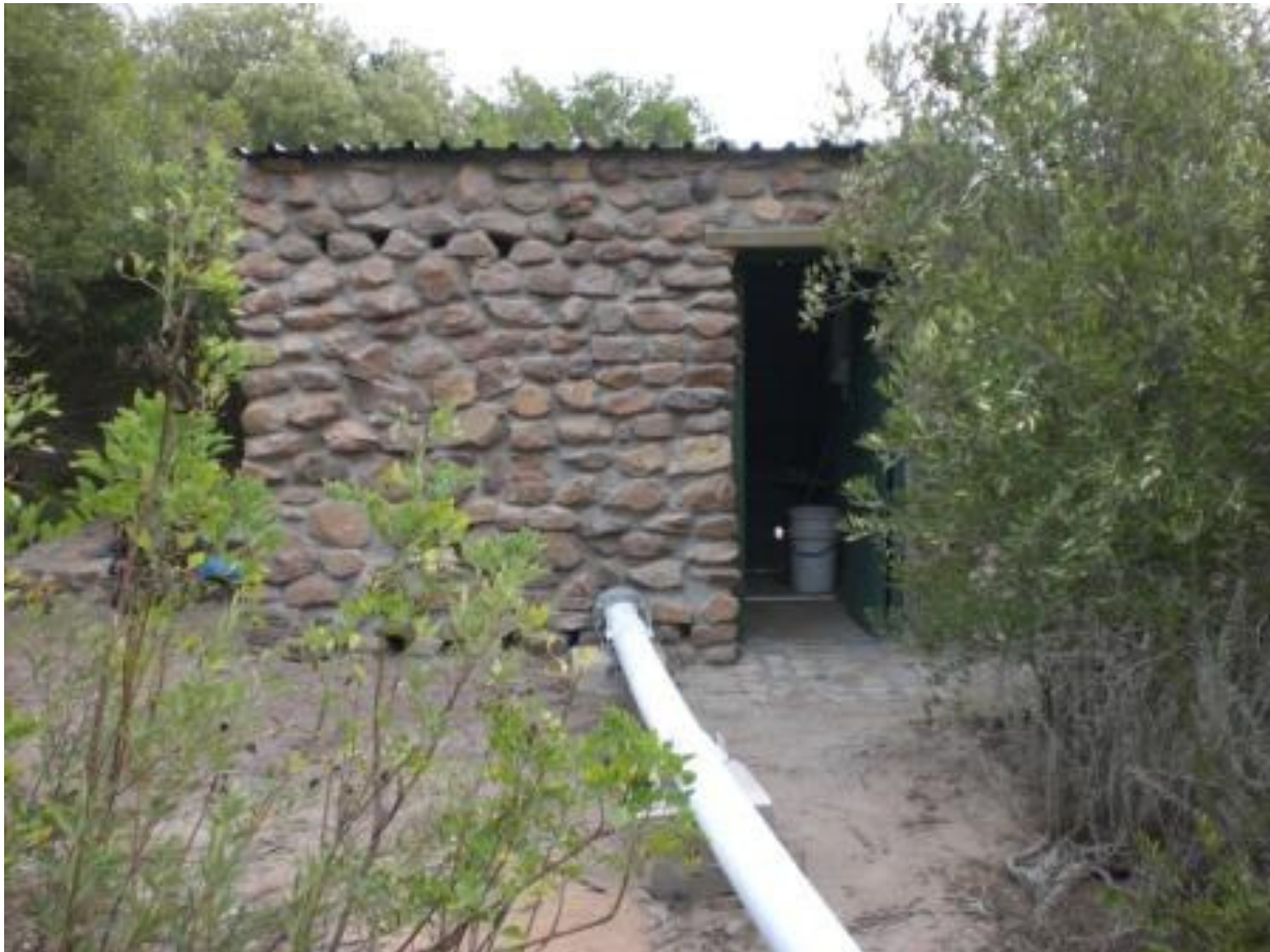
Figure G.5: The powerhouse from the front where the main pipeline enters.
