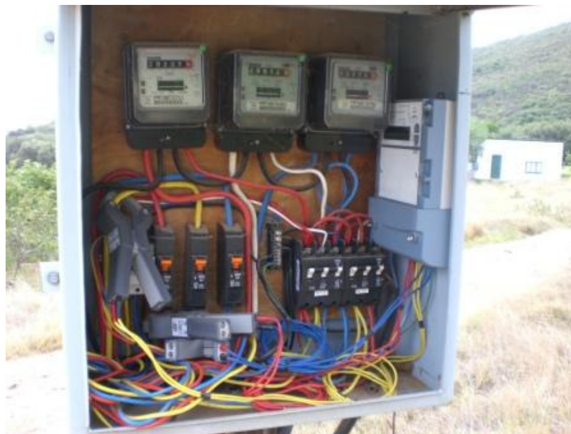
Figure G.16: Main distribution board where the MHPS is connected to the load and grid.
