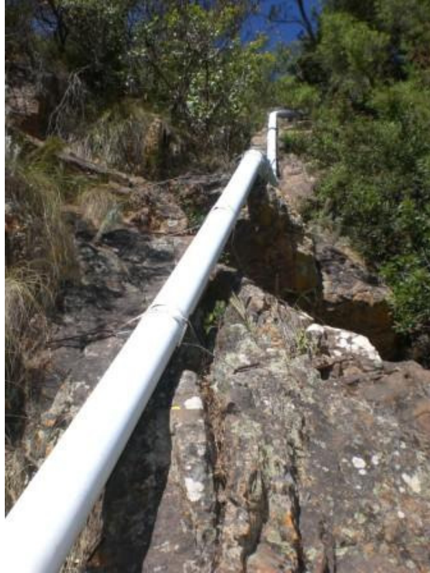
Figure G.9: Part of the above ground pipeline with the constructions that holds the pipes to the boulders.
