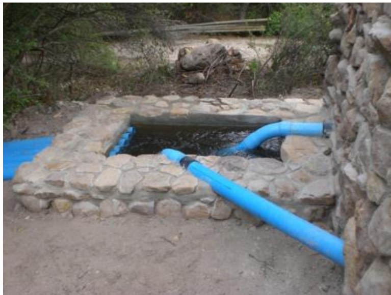
Figure G.14: Tailrace dam with the bypass line in the lower right corner and the draft tube in the middle.
