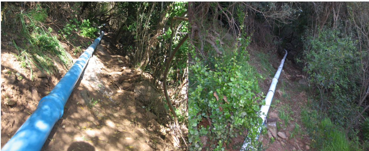
Figure G.18: The above-ground part of the pipeline, just after installation (on the left) and after a year (on the right)
