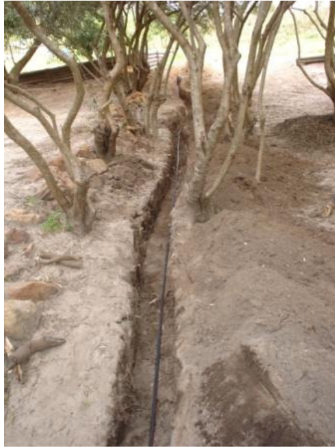
Figure G.11: Power cable trench with the cable lying in it.
