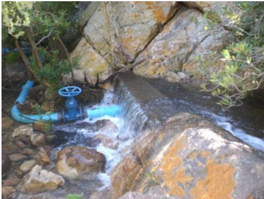
Figure G.10: The isolation valve and pipeline constructed into the diversion weir, with the trash rack located behind the diversion weir.
