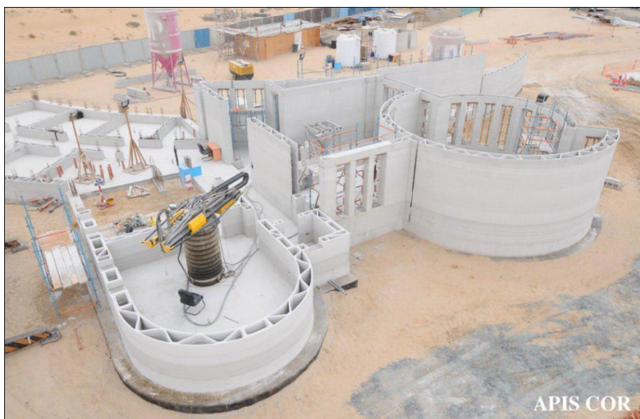
Figure 2.3: Construction of a Two-Storey Office in Dubai Using 3D Printing Technology by Apis Cor.
