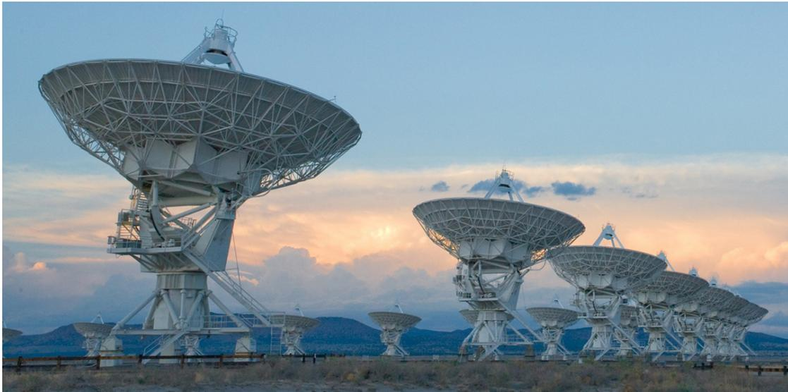
Figure 2.2: The VLA located in Socorro, USA, is an example of an array telescope, consisting of 27 radio antennas. Each antenna in the array measures 25 meters (82 feet) in diameter and weighs about 230 tons.
