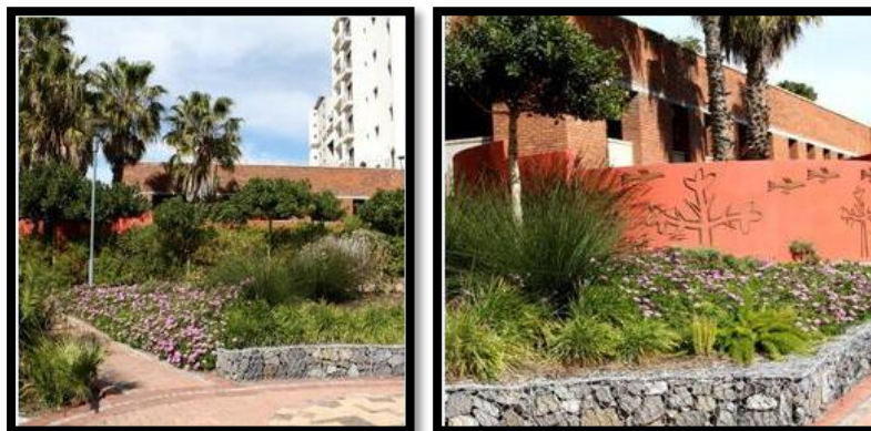
Figure 13: Combined techniques in Century City used for drainage prior to conveyance to the wetlands
