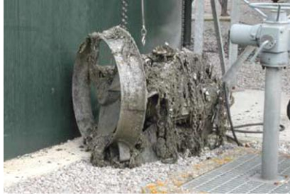
Figure 2.12: Damaged horizontal paddle stirrer (from CAE, 2012).
