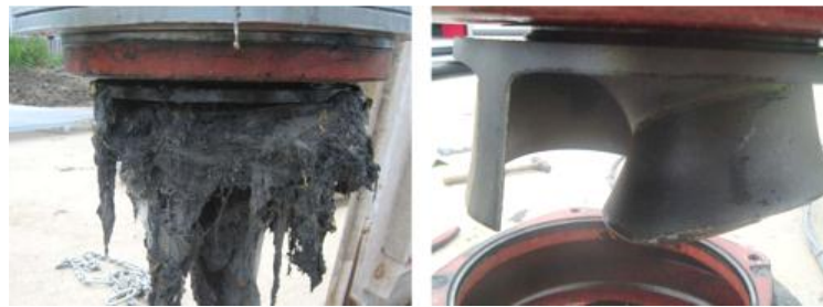
Figure 2.13: Blockage of a slurry-recirculation pump for a digester mixing system: a) before and b) after cleaning (from CAE, 2012).
