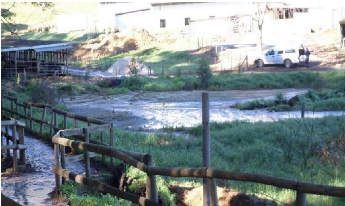
Plate 4: A constructed wetland to manage dairy manure wastewater at Welgevallen experimental farm
