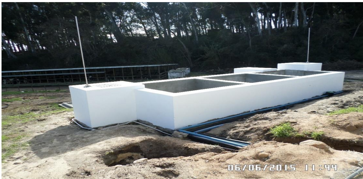
Plate 7: Three chamber, plug-flow anaerobic reactor at Welgevallen experimental farm.
