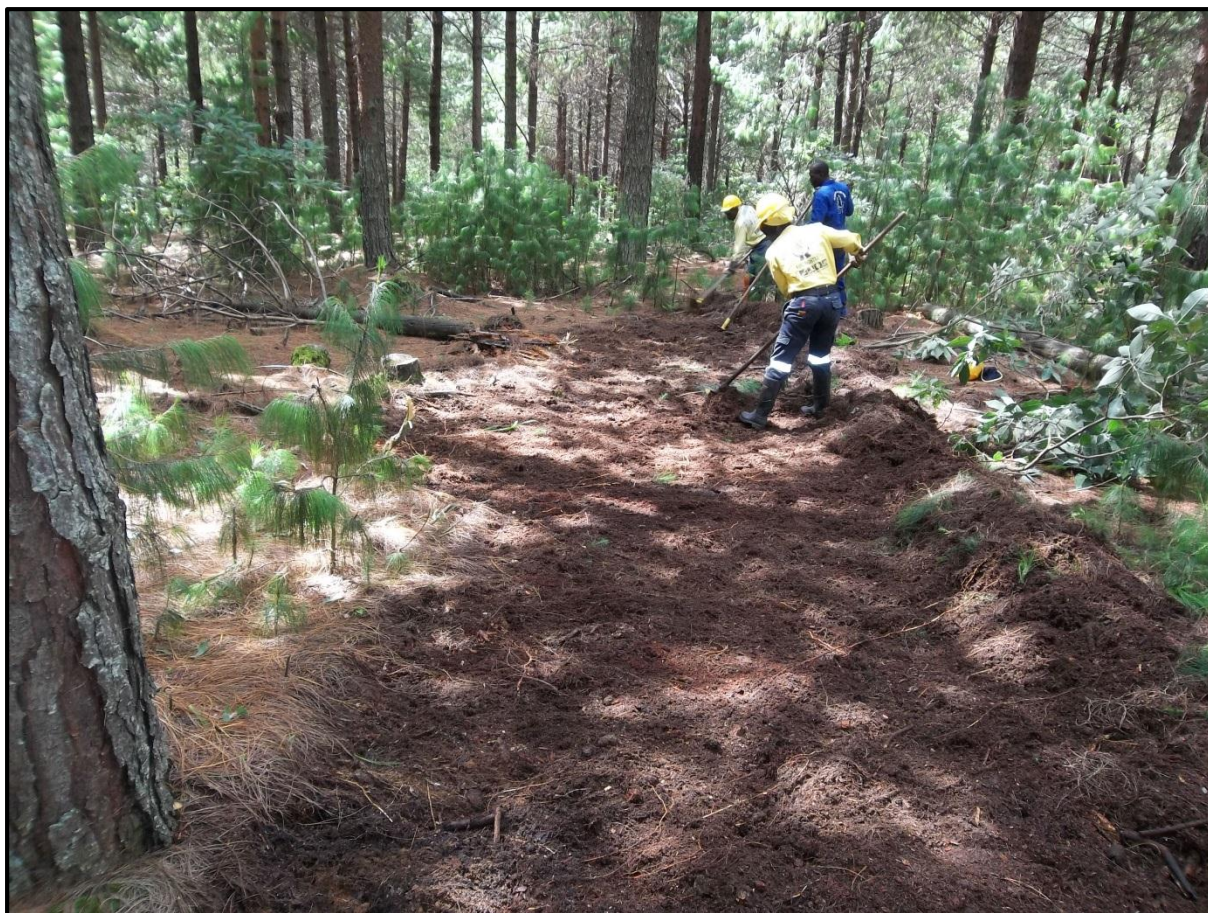
Figure 3.10: The construction of the fire breaks using rake hoes to remove all flammable material.
