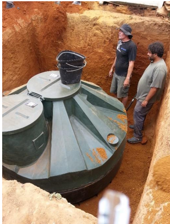
Figure 3.10 The Biogaspro anaerobic digester at Enkanini
