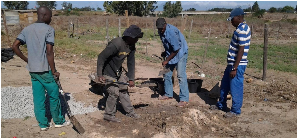
Figure 3.11 Klipheuwel residents involved in the construction of the pour-flush toilets
