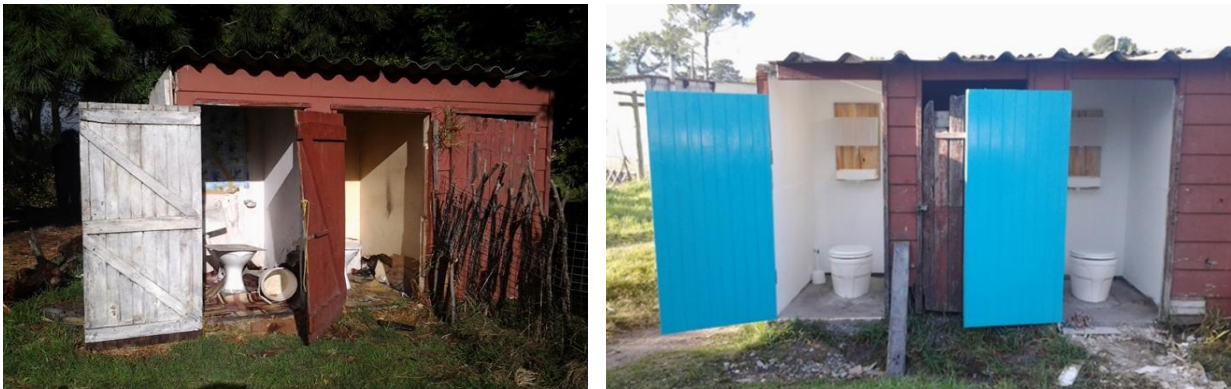
Figure 3.3 From left to right: Two previously broken down toilets replaced by the pour-flush toilets (Author, 2013)
