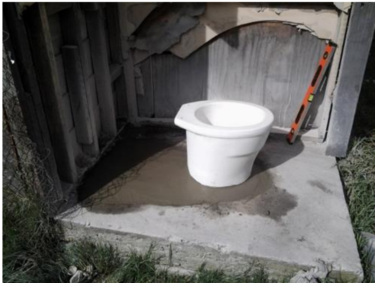
Figure 3.8 Pour-flush pedestal and P-trap design (source: Maluti GSM, 2014)
