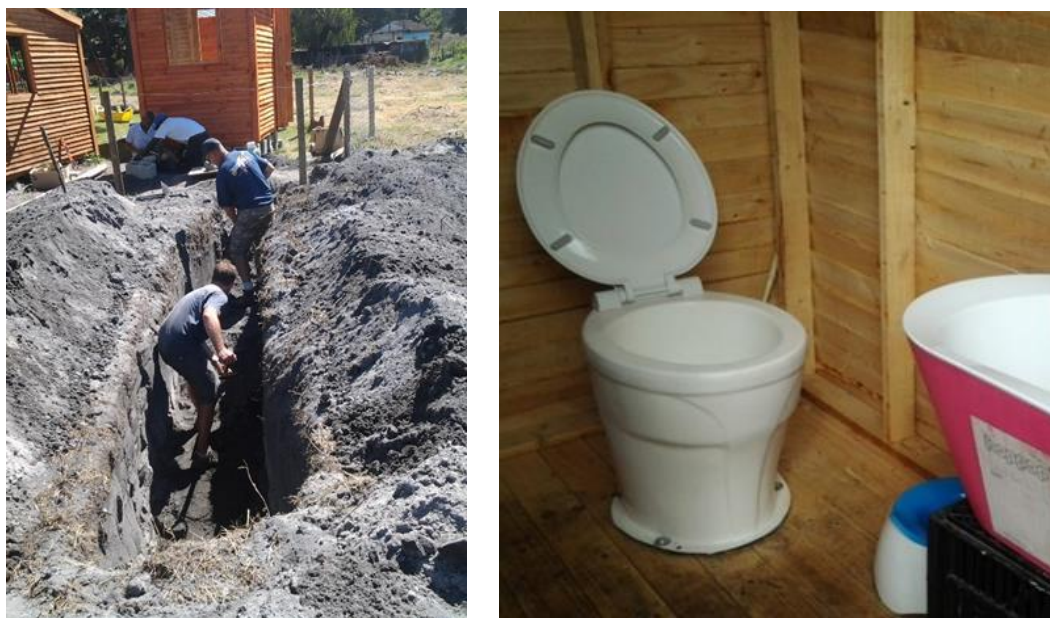
Figure 3.4 From left to right: Installations at the crèche and the crèche toilet (Author, 2013)
