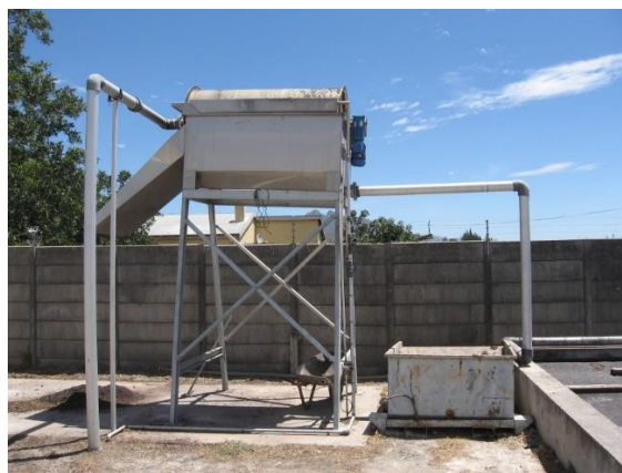
Figure 2.4. Screening equipment used to remove coarse particles from the winery wastewater.
