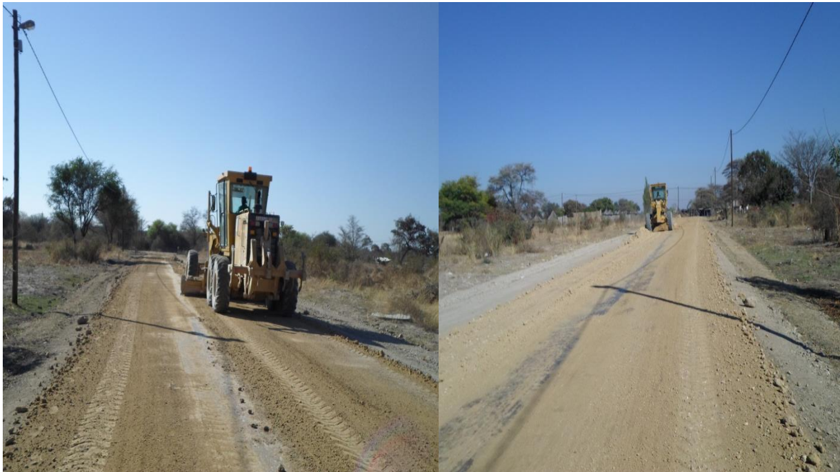
Figure 18 Streets under construction
