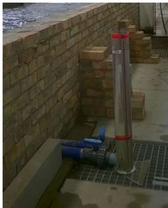
Figure 3-6. Tailwater gauge (manometer) for measuring the tailwater depth
