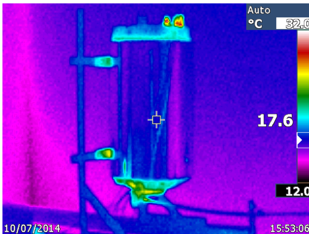
Figure 4-19: Water heater B (vertical), thermal image of the water heater.
