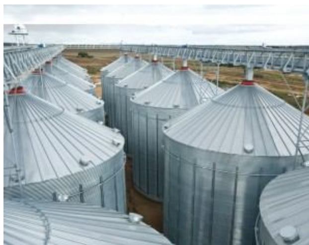
Figure 2.7: Typical bins on bulk production and storage plants
