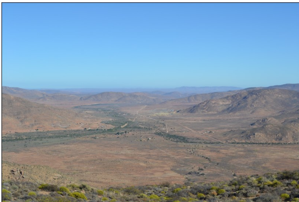
Figure 3: The view looking from the inland plateau down the river catchment. The town of Buffelriver is just to the left.
