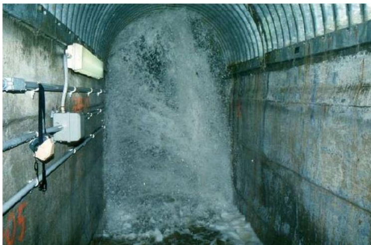
Figure 1-1 Water leaking into a gallery from a crack at Upper Stillwater Dam (Hansen & Forbes, 2012).
