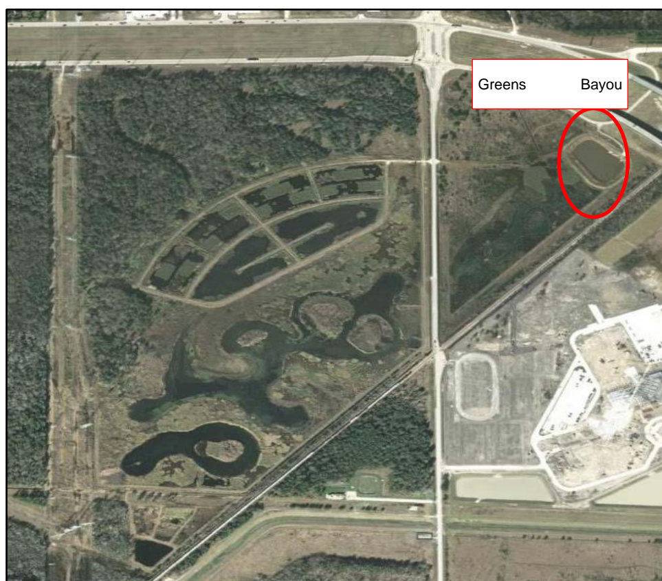
Figure B-9 Greens Bayou retention pond located on the Beltway 8 Wetland Water Quality Project (Wetland Solutions Inc., 2010)
