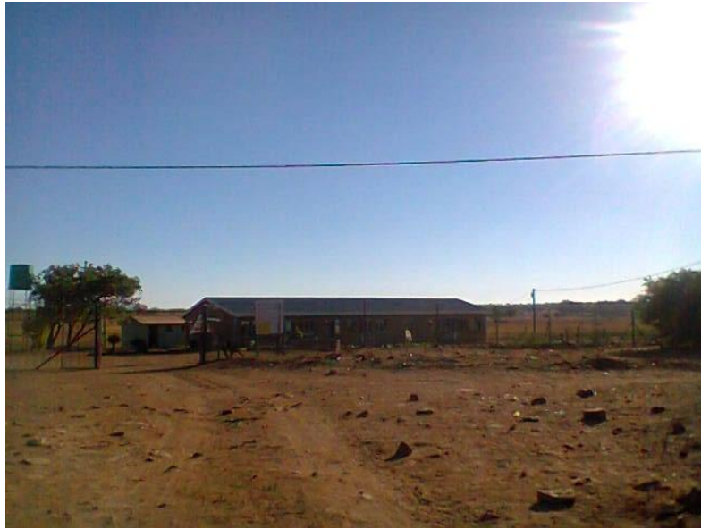
Figure 5.1: The external view of Site A
