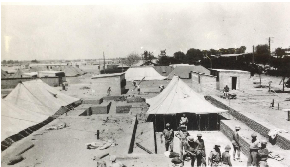
FIGURE 3.5: Construction of a General Hospital 87
