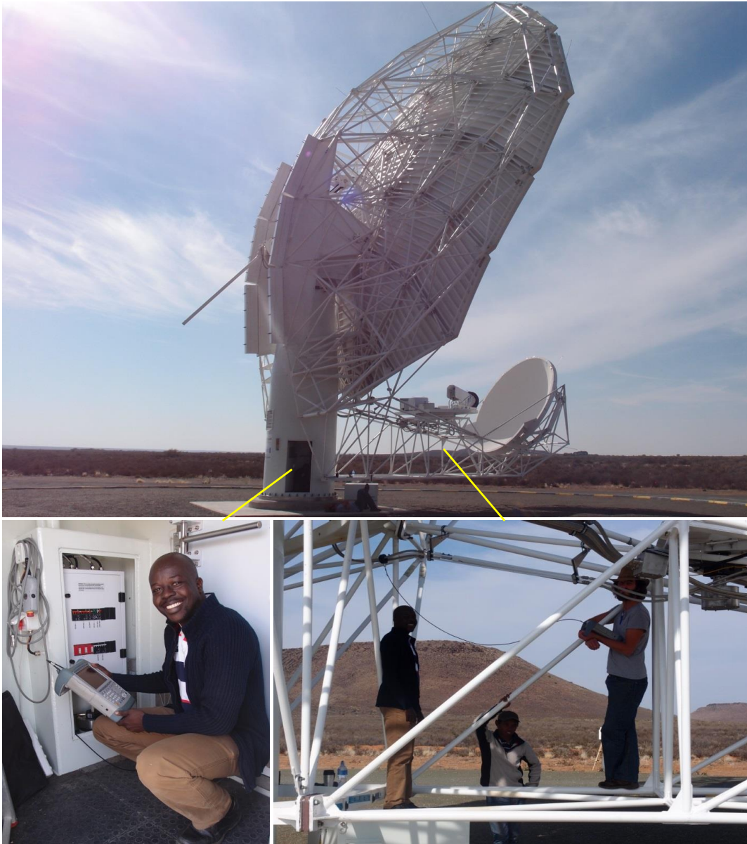
Figure 4.3: Top: Full MeerKAT dish with pedestal door opened. Bottom left: Measurement of induced currents on the earth stub-up within the pedestal. Bottom right: Measurement of RF levels on the cables below the RI using current probe and spectrum analyser.
