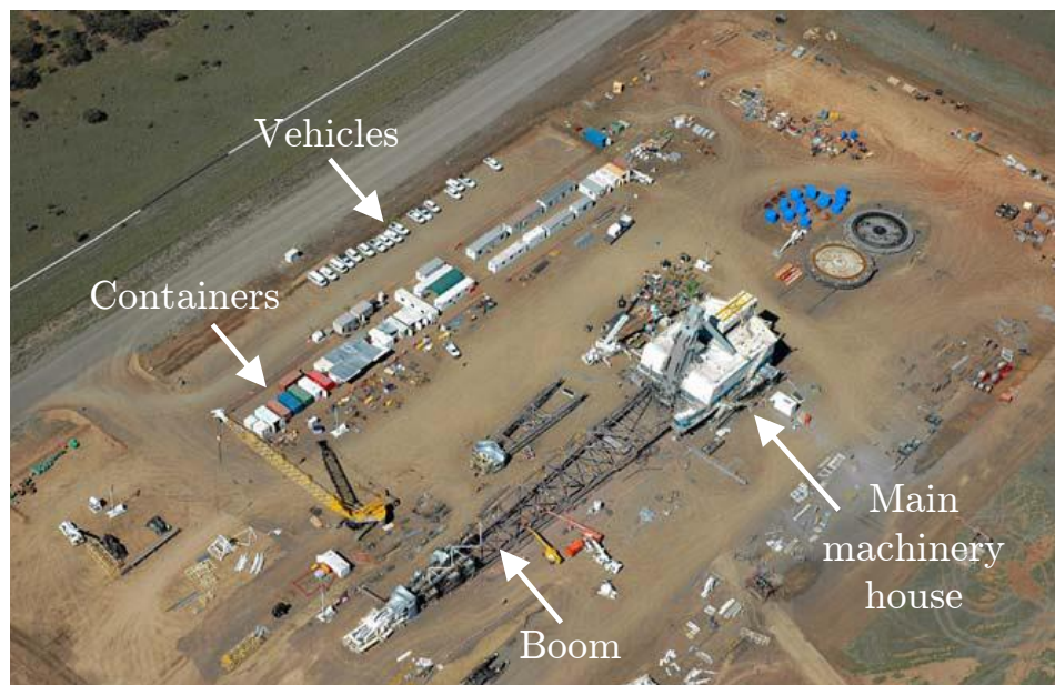
Figure 5.4: Aerial view of a dragline shutdown site
