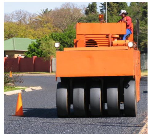
Figure 4: Roller compaction in seal construction (van Zyl, 2015)
