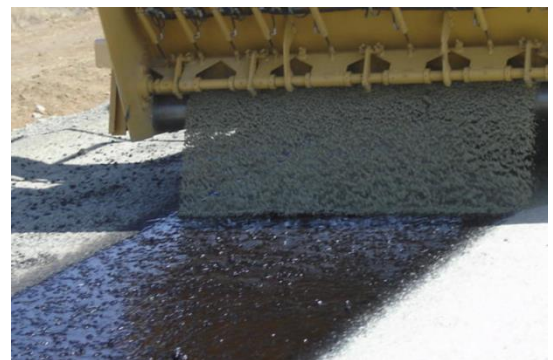
Figure 33: Aggregate application in seal construction practice (van Zyl, 2015)
