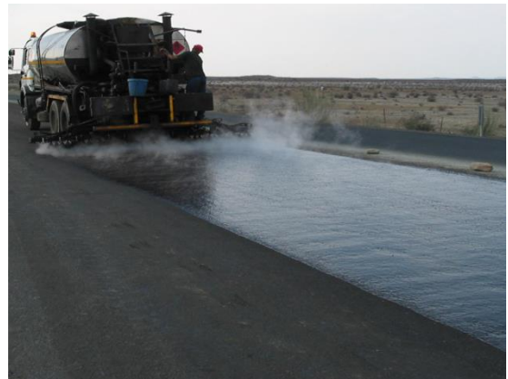
Figure 32: Tack coat application in seal construction (van Zyl, 2015)
