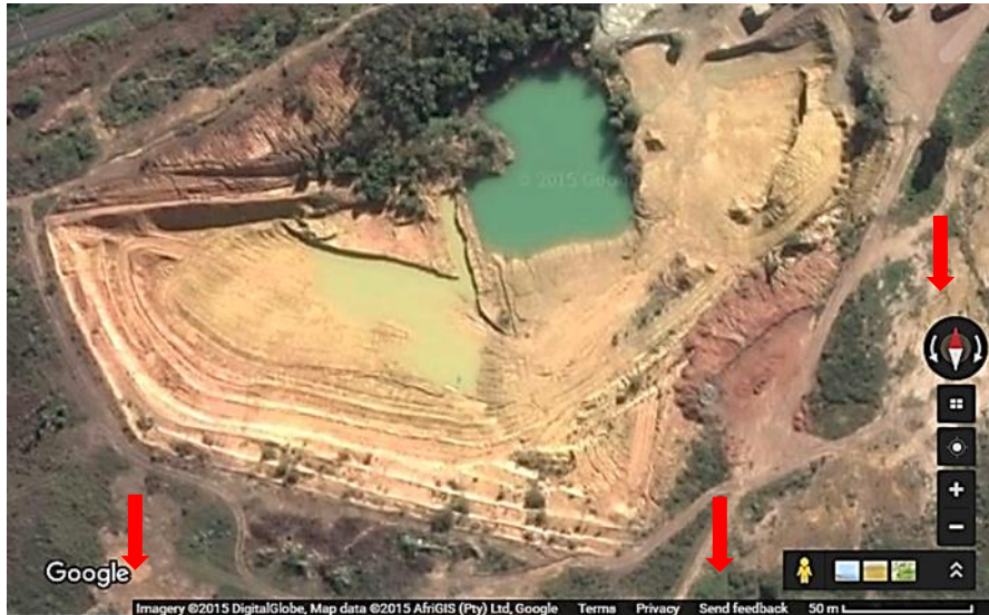
Figure 3-11: An aerial photograph of Boland Bricks, Contractor Rd, Courtrai, Paarl (courtesy, Google imagery).
