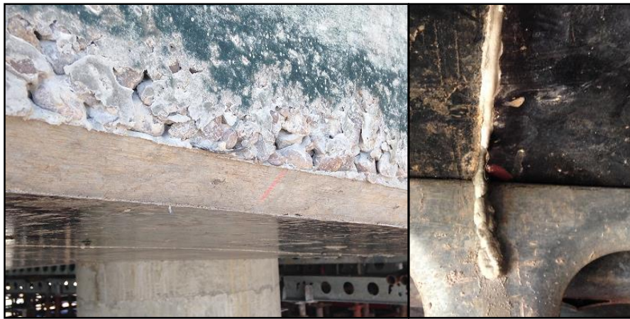
Figure 18: Possible SCC impacts on construction (Left: Poor NCC concrete compaction in the formwork corners, Right: Formwork leakage at a shutter connection underneath a bridge deck slab)
