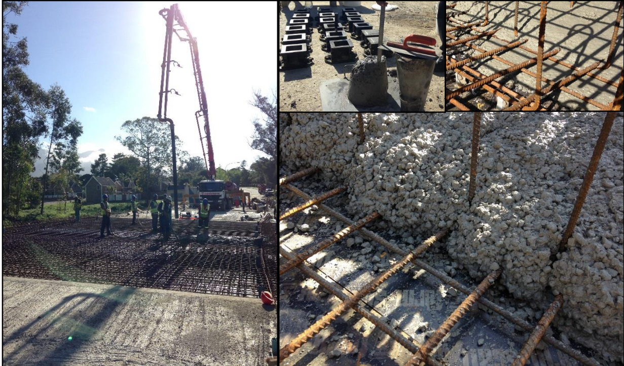
Figure 17: On-site construction activities (Left: Concrete placement by pump, Top middle: Regular slump test, Bottom right: Fresh concrete after pump discharge, Top right: Fresh concrete after vibration)
